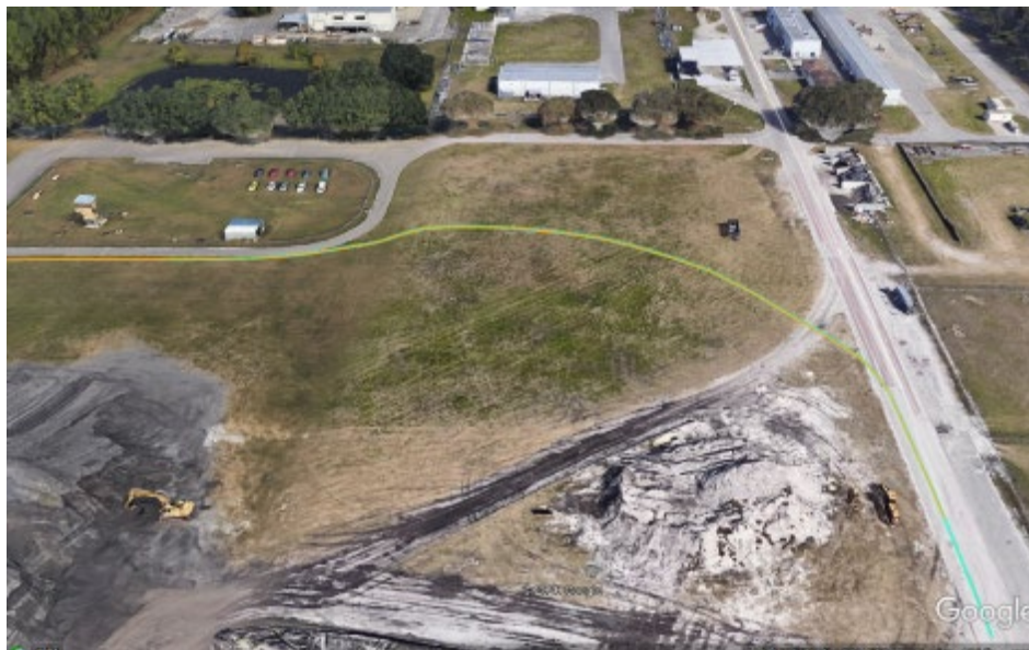
Figure 6-67. The trajectory of the vehicle from the pavement to the grass for Test Case 11
