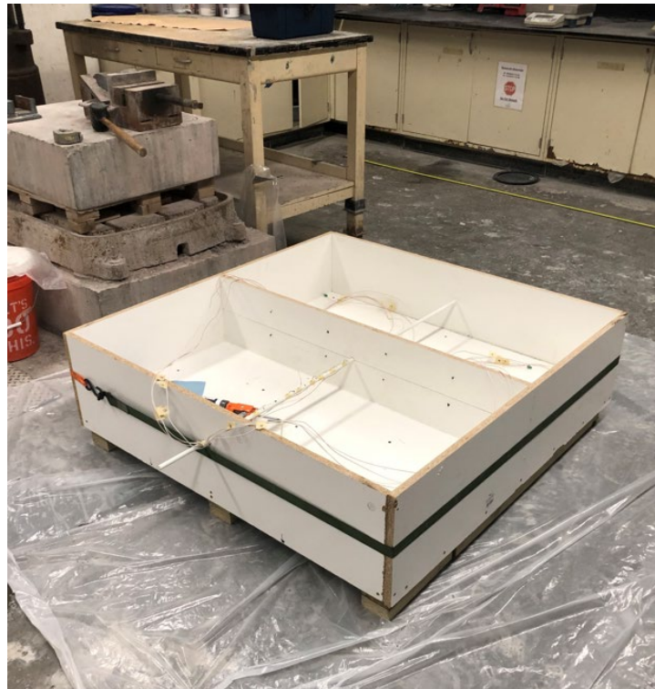
Figure 51: Formwork for slabs construction
