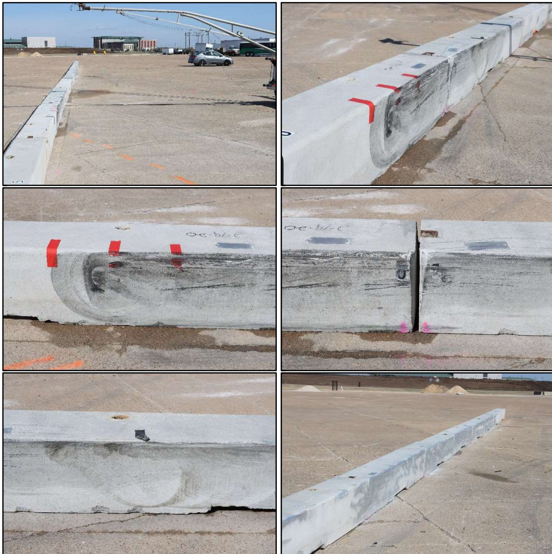
Figure 5.3. Portable Concrete Construction Zone Barrier after Test No. 690905-UOF1.
