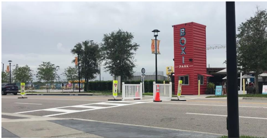
Figure 6-4. EB left-turn bay blocked using fences
