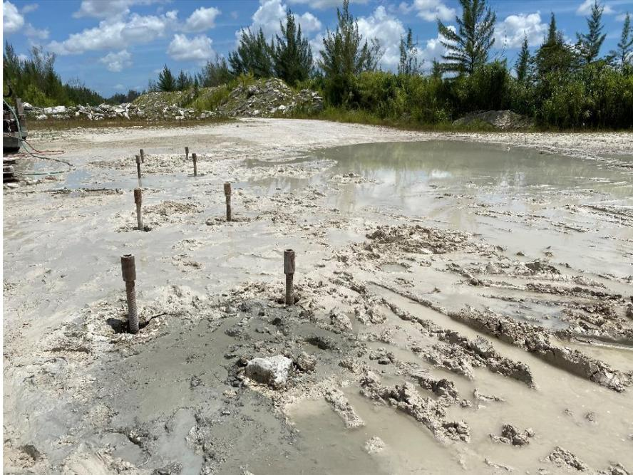
**Figure 5-17 Eight micropiles after installation**
