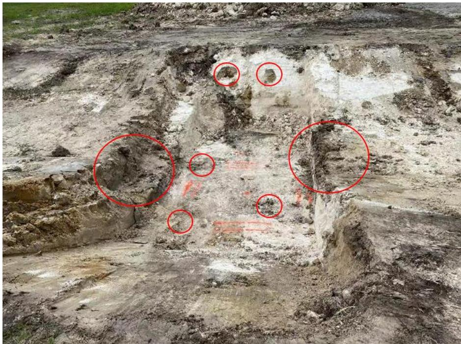
**Figure 7-13. Footing location excavation (circles identify soil-filled voids)**
