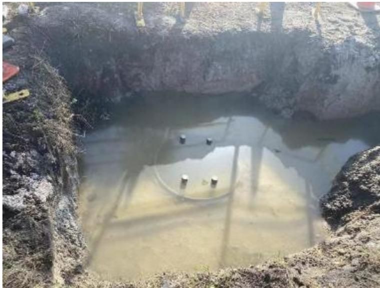
**Figure 6-22 Picture of the east drilled shaft after two days of installation**
