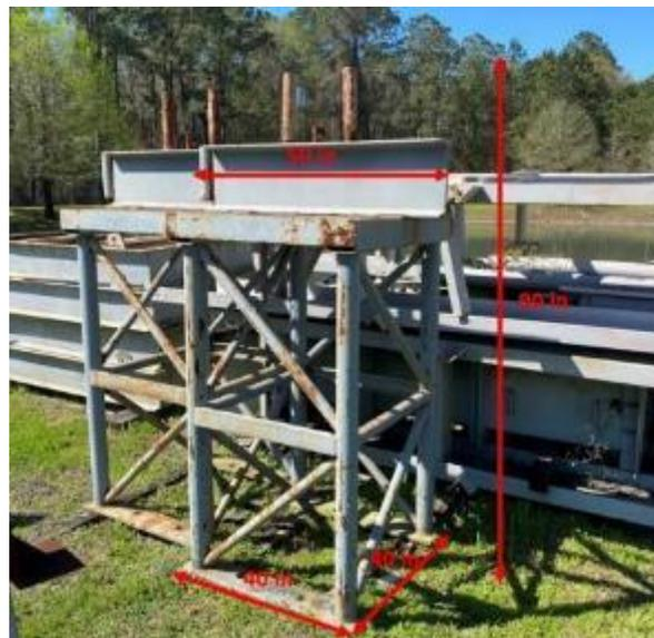
**Figure 6-25 Stands to support the girders**
