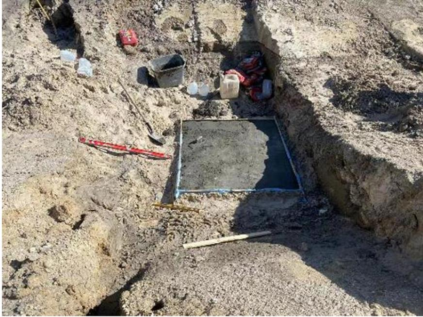
**Figure 7-14. One in concrete leveling pad for placement of the steel foundation elements**
