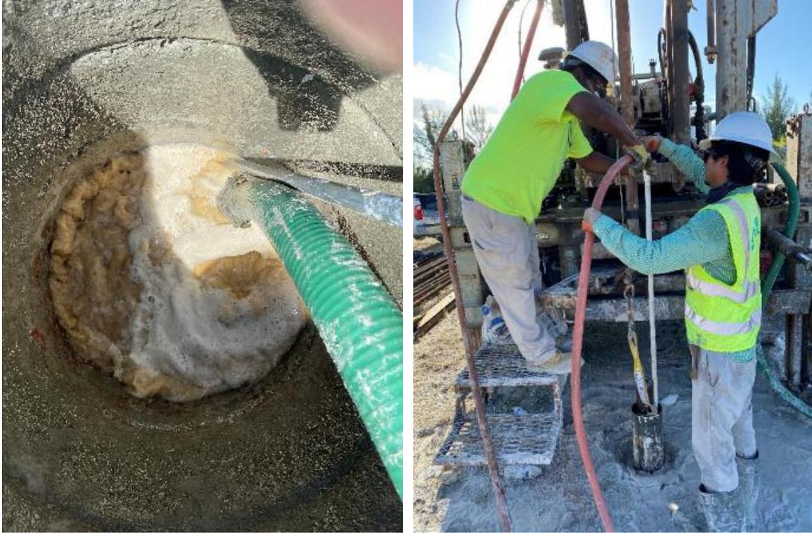
**Figure 5-15 Grouting process (the grout mixed with ASTM C494 Type D retarder admixture and the ASTM C494 Type F superplasticizer admixture)**
