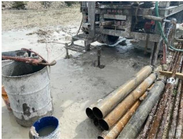
**Figure 5-9 6 in casing used for drilling**
