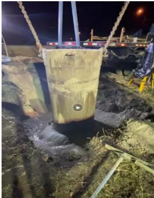
**Figure 6-21 Temporary casing pull out and concrete overflow**
