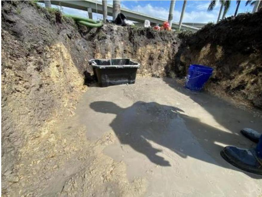
**Figure 6-26 Fast setting concrete placement**
