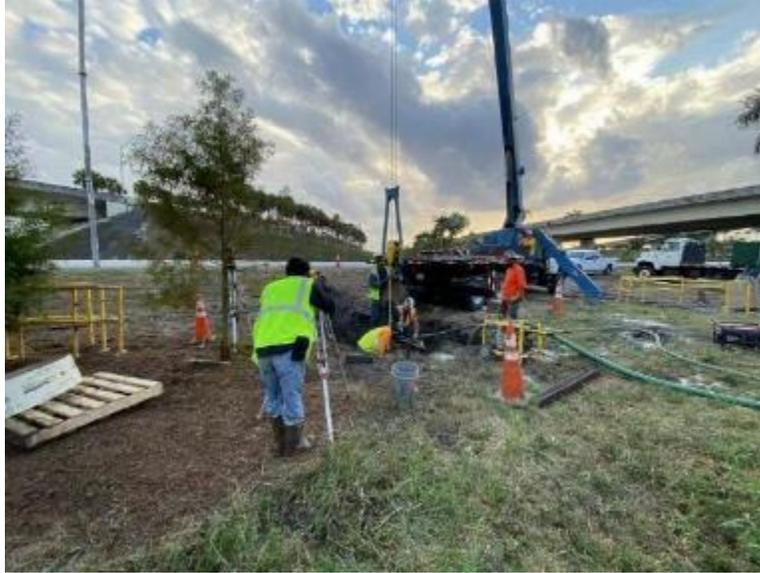
**Figure 6-19 Measure the depth of the top of the threaded rods (2 ft from the ground surface) and align the drilled shafts**
