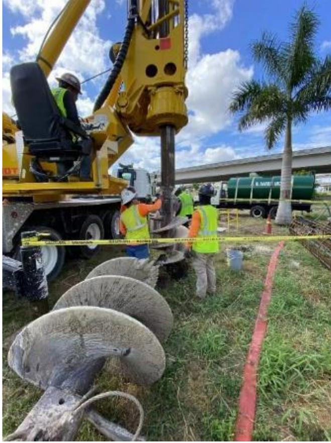
**Figure 6-16 Change to the 36-in rock auger bit**
