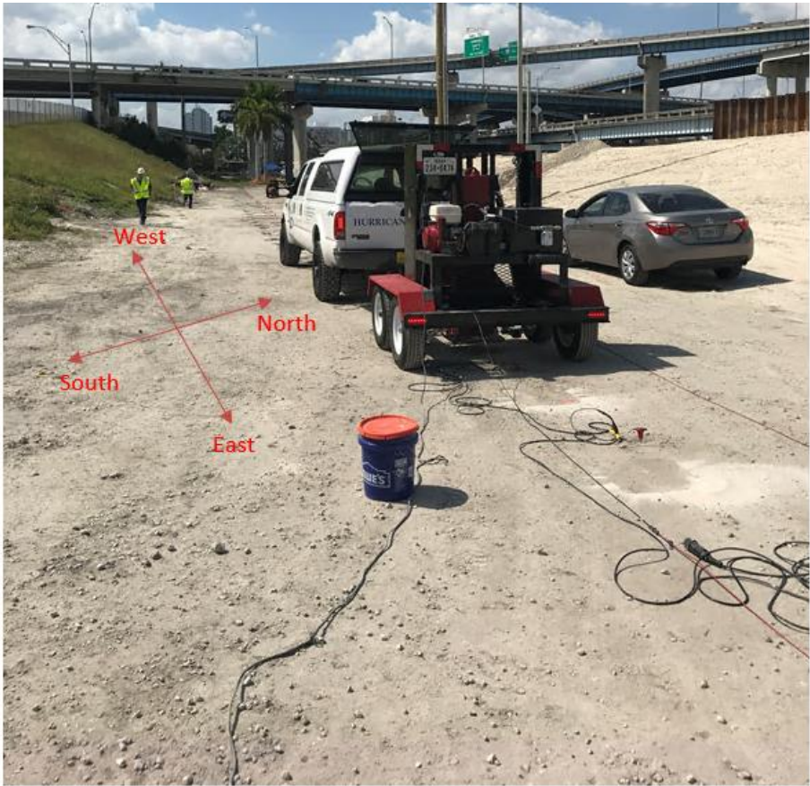
Figure 4.14. Miami test site
