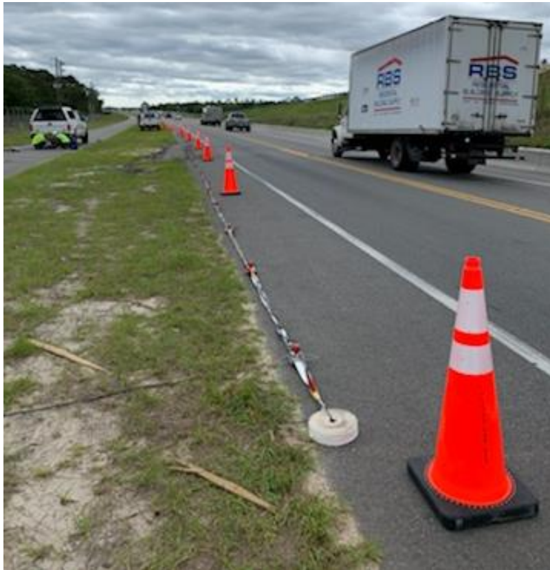
Figure 4.20. Wekiva Parkway SR-46 site with a known sinkhole
