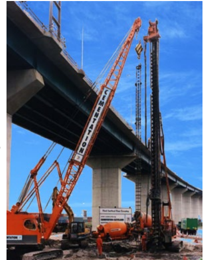
ACIP piles at a bridge interchange.
