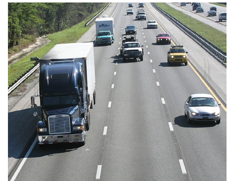
Efficient roadways and timely delivery are critical factors for millions of tons of freight moving on Florida roadways every day.
