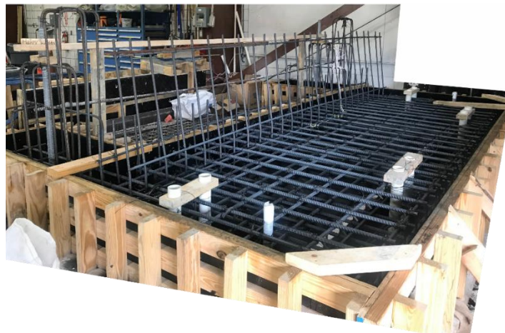
Figure 7-1 Reinforcing bars positioned inside deck formwork for steel reinforced specimens
