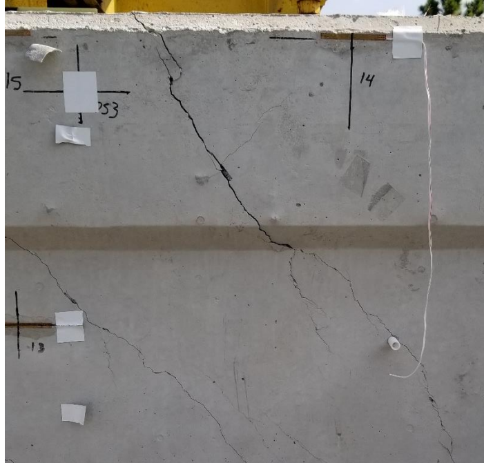
Figure 9-25 Crack on the back face of GFRP EOR-1 specimen with width wider than 0.10 in.
