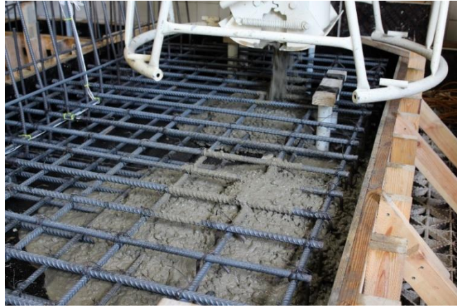
Figure 7-4 Deck concrete placement
