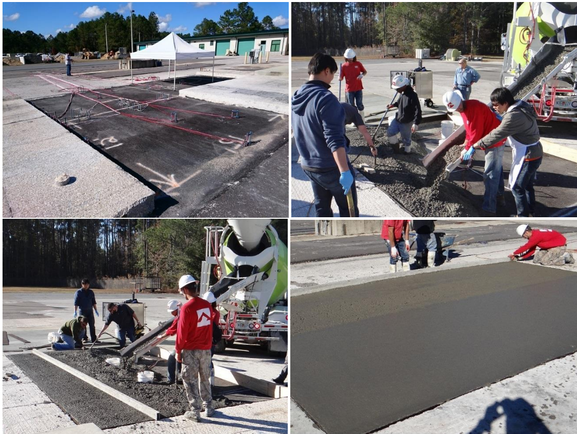
Figure 5-1. Construction of an APT test slab.
