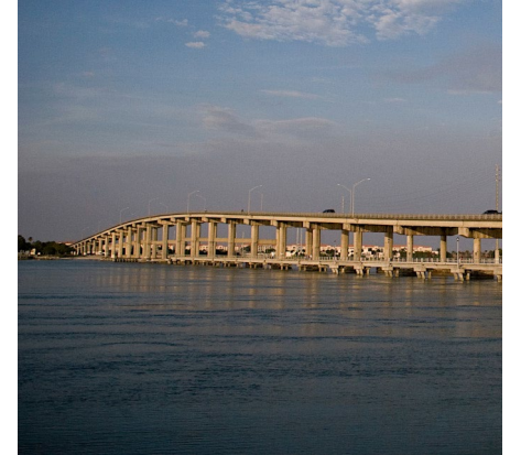
Florida bridges, both large and small, must be built on foundations that take into account Florida's highly variable soils.
