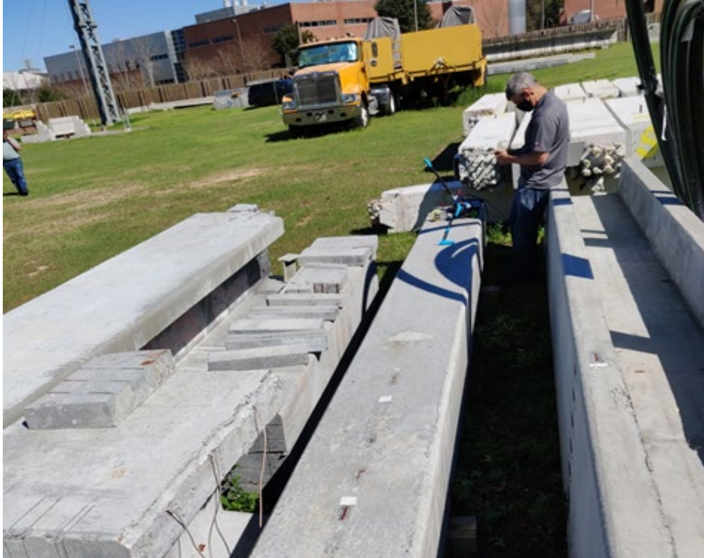
Figure 227: Square pile during scanning
