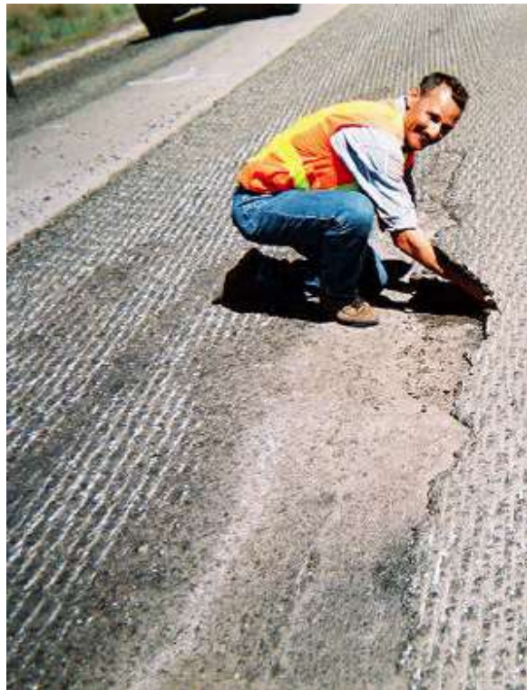
(b) Milled surface of SR 97A
