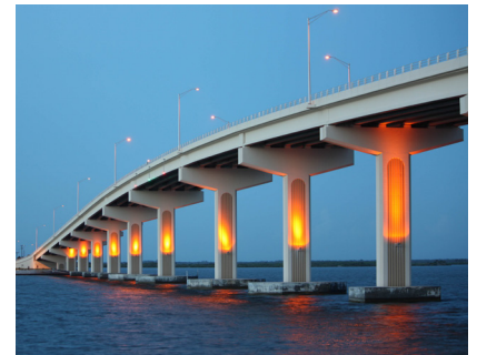
Prestressing allows concrete girders to be longer, lighter, and stronger, saving time.
