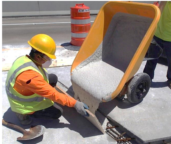
Figure 2-1 UHPC used for joints of deck panels
