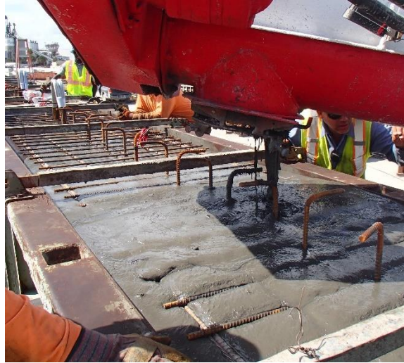
Figure 2-2 UHPC used to fabricate prestressed girders
