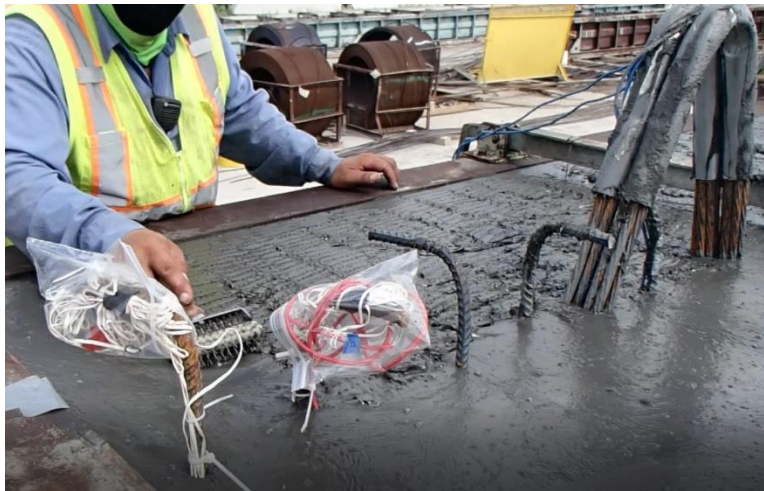
Figure 3-16 UHPC surface finishing
