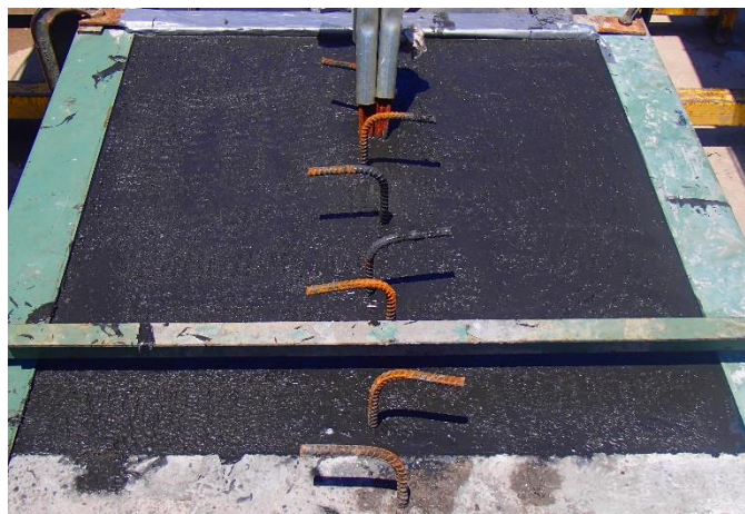
Figure 4-9 Finalized UHPC section at girder end
