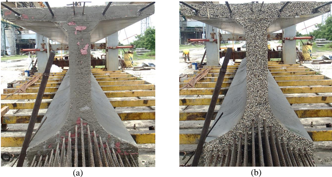
Figure 4-7 SCC surface preparation: (a) Prior to water jetting and (b) After water jetting
