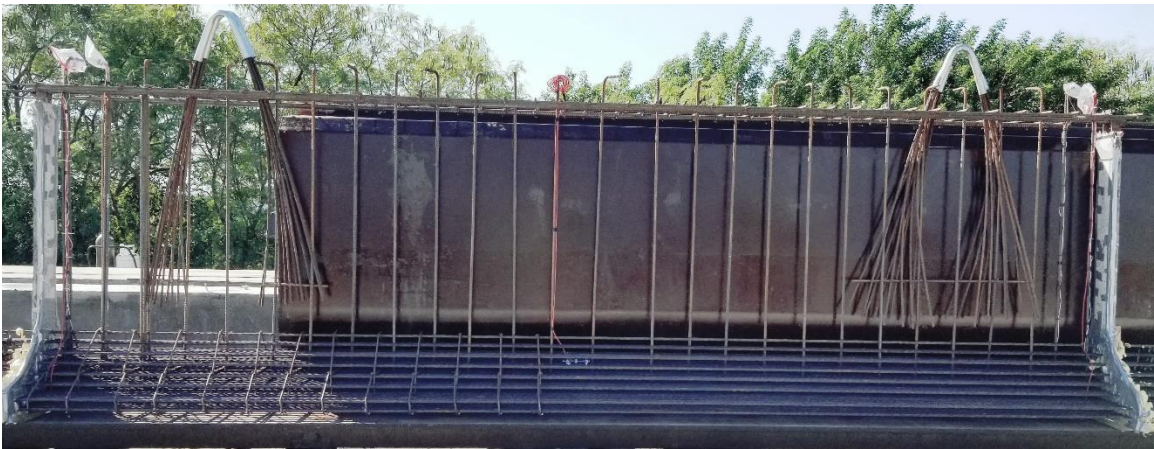
Figure 3-8 Mild-steel reinforcement in G4
