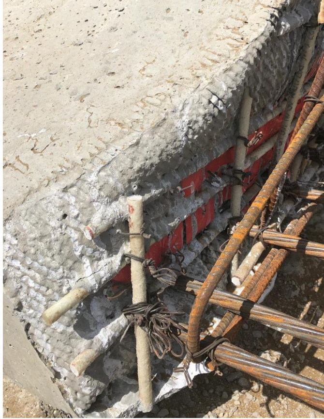
Figure E-5 Mesh surface after concrete pour
