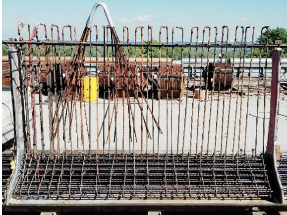
Figure 3-5 Mild-steel reinforcement in SCC portion of G1
