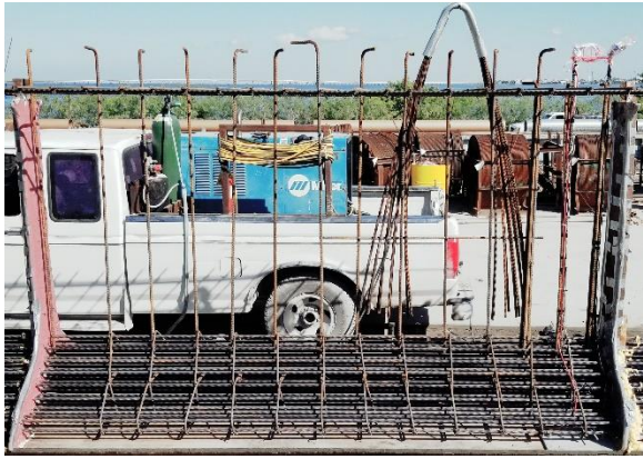
Figure 3-6 Mild-steel reinforcement in SCC portion of G2
