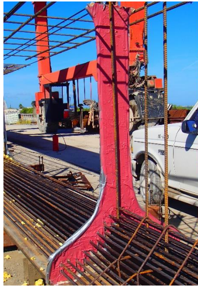
Figure 3-10 Application of concrete retarder admixture to bulkhead
