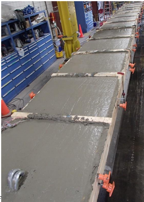
Figure 4-27 Finished deck construction
