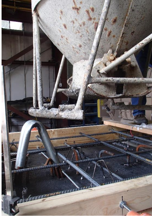
Figure 4-26 Method for concrete placement
