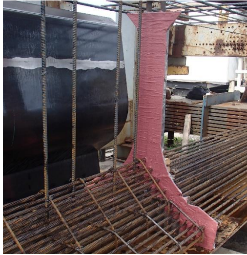
Figure 4-6 Application of concrete retarder on bulkheads
