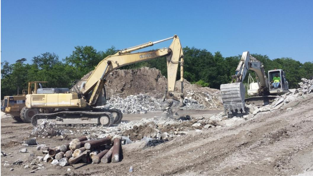
**Figure 22:** Concrete being crushed at Florida Concrete Recycling facility in Gainesville, FL
