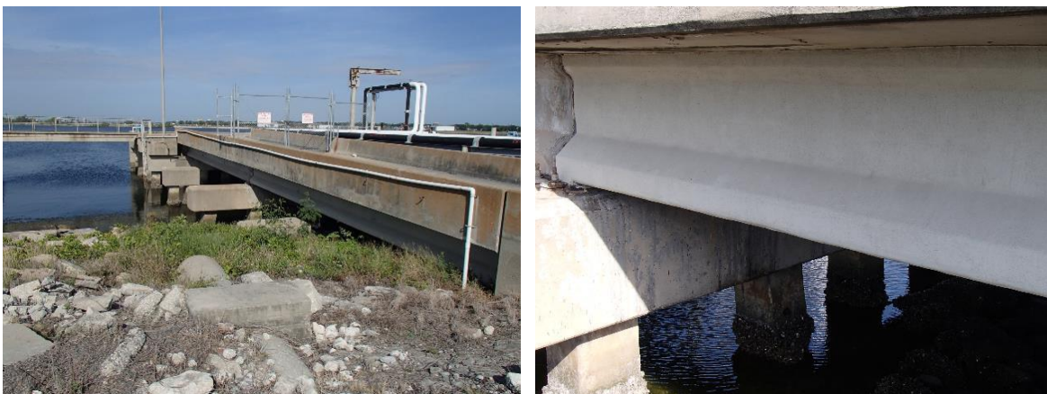
Figure 63—Site conditions at Port of Tampa Berth 21
