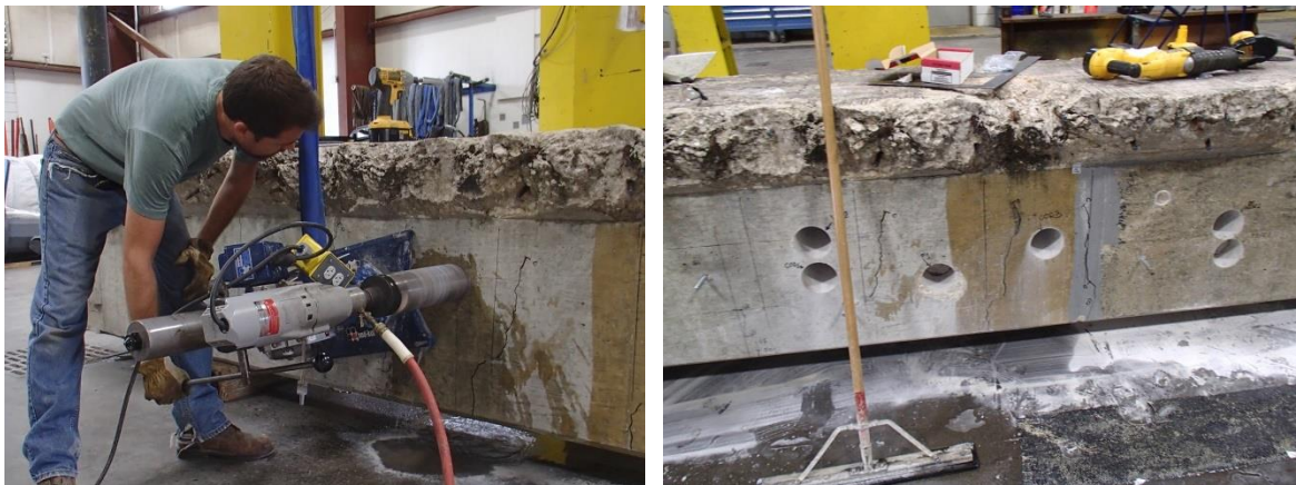
Figure 92—Coring of bridge girders
