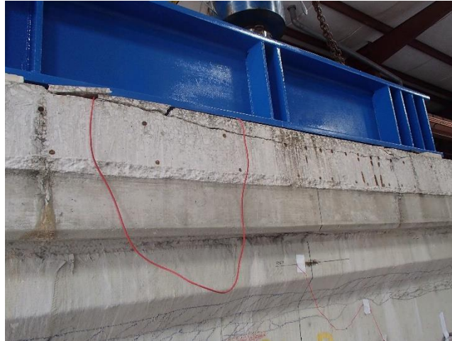
Figure 250—Concrete crushing in the compression zone
