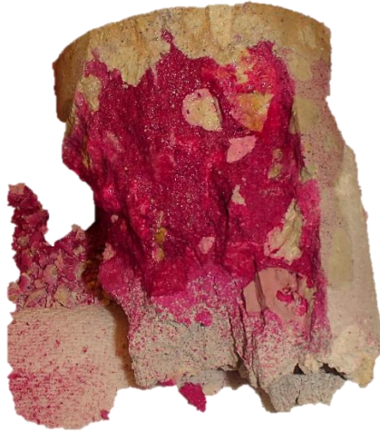
Figure 95—Concrete carbonation examined on a concrete cylinder following the compression test
