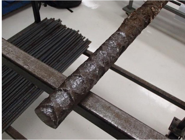
Figure 144—Reinforcement with bare metal exposed
