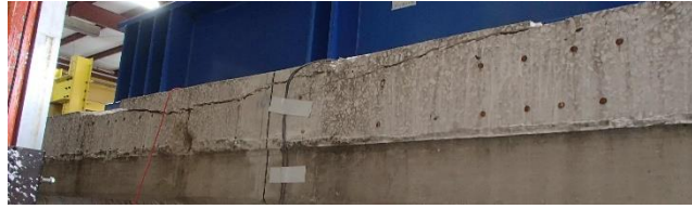
Figure 246—Concrete crushing in compression zone
