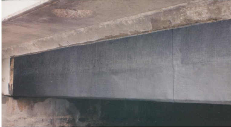
Figure 82—Exterior Indian River Bridge girder wrapped with bidirectional CFRP
