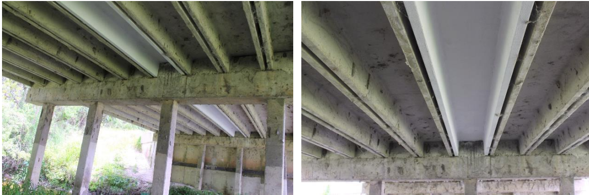
Figure 71—Repaired superstructure on Durant Road Bridge
