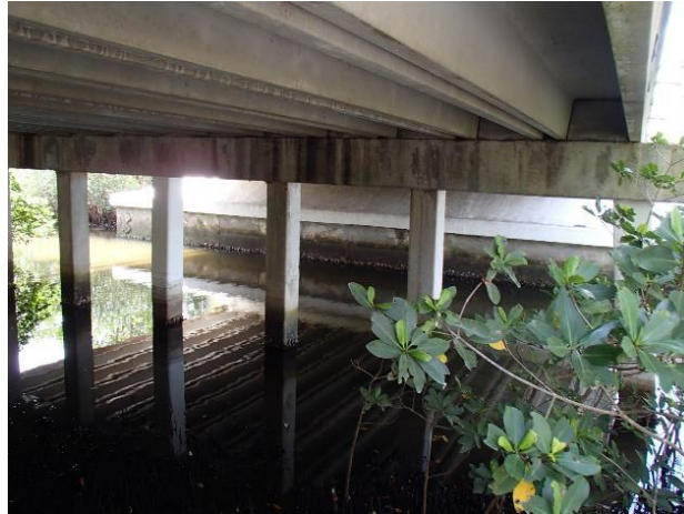
Figure 67—Repaired piles on Dickman Road Bridge
