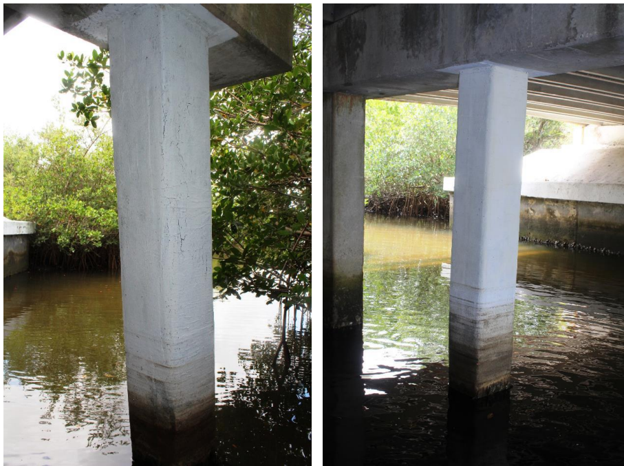
Figure 68—FRP-confined piles on Dickman Road Bridge
