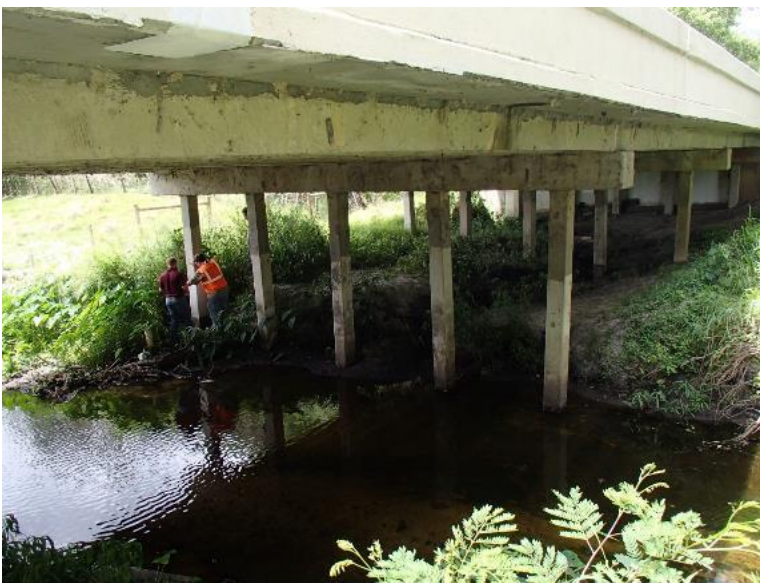
Figure 70—FRP-confined pile on Durant Road Bridge
