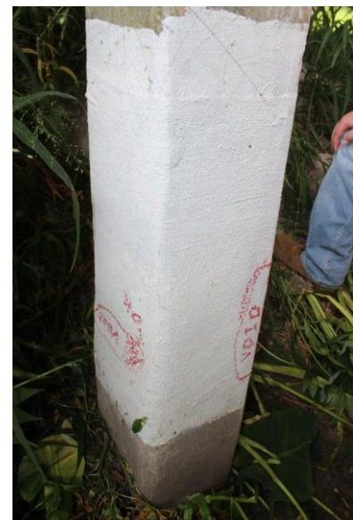
Figure 70—FRP-confined pile on Durant Road Bridge
