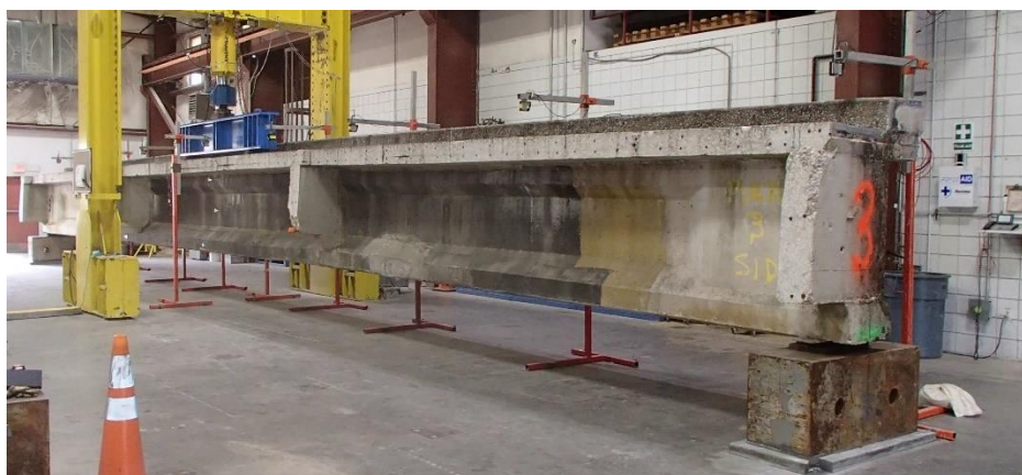
Figure 238—Girder loaded in test frame
