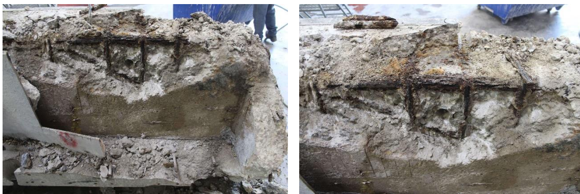
Figure 220—Corroded steel reinforcement in the north end of Girder 3-1
