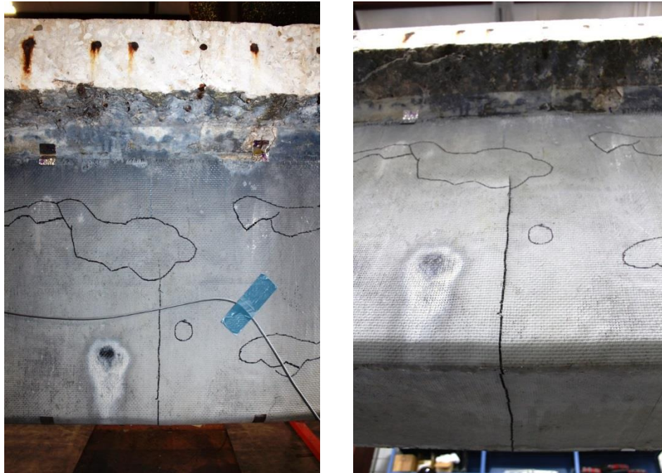
Figure 113—Rupture of CFRP near midspan
