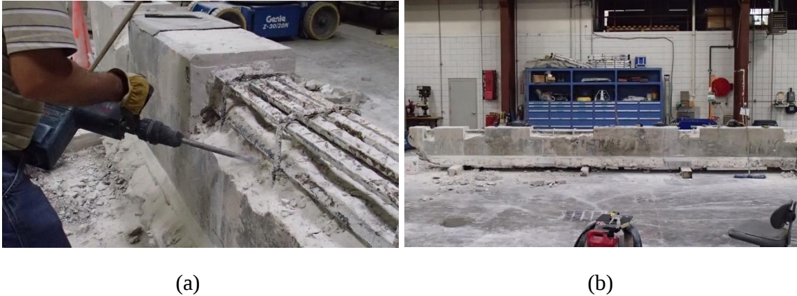
Figure 124—(a) Chiseling of concrete surrounding the reinforcing bars and (b) bridge girder in upside-down position
