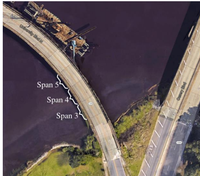
Figure 132—Aerial view of the University Boulevard bridge
