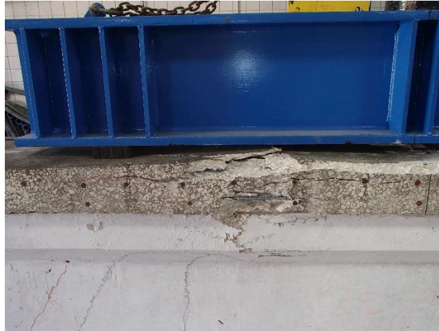
Figure 252—Concrete crushing in the compression zone
