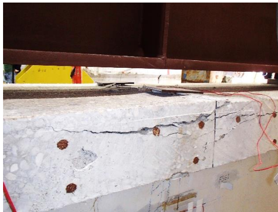
Figure 190—Crushing of concrete in compression (east elevation view of Girder 3-2)
