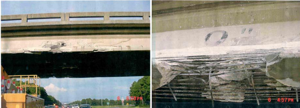
Figure 227—Girder damage from vehicle impact in July of 2001
