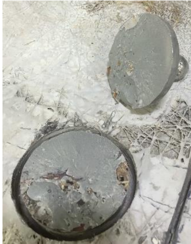
Figure 155—Smooth dolly that failed at the dolly-to-FRP interface
