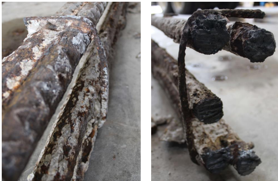
Figure 145—Steel reinforcement welded together with stirrups
