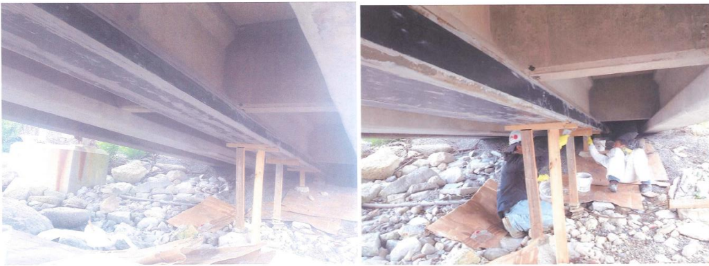
Figure 62—CFRP laminate strip installation at Port of Tampa Berth 21
