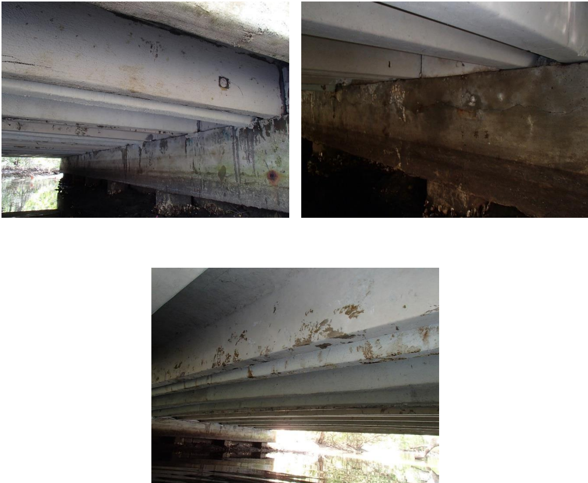
Figure 64—Girders with external FRP on Phillips Lane Bridge
