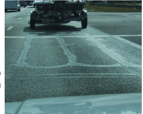
These familiar pavement marks indicate the presence of inductive loop detectors, which collect data as vehicles pass over them.
