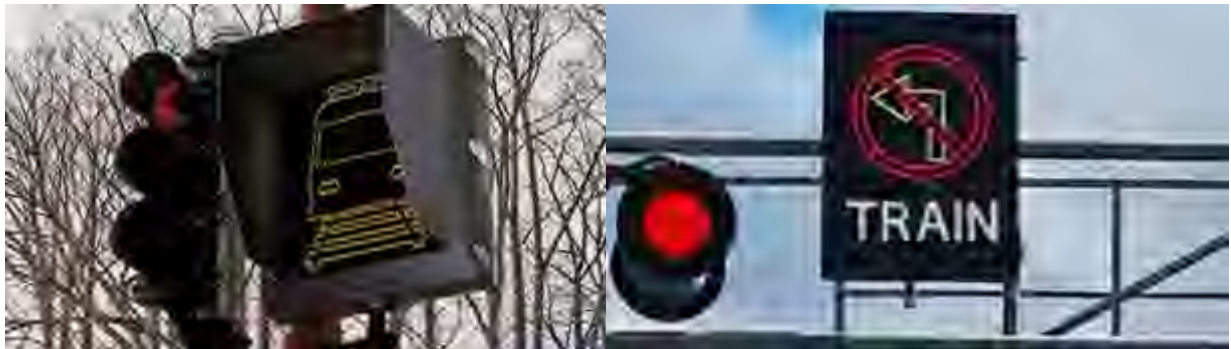
Figure 40 Examples of a LED preemptive train warning sign.
