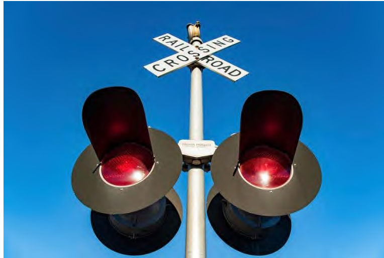
Figure 38 An example of flashing light signals. Source: Klassy. (2017). Railroad Crossing Lights
