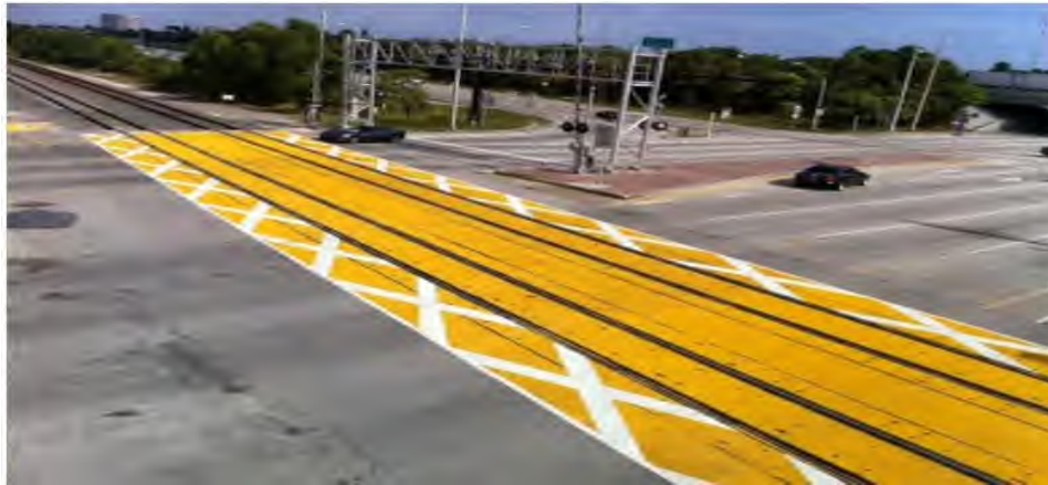
Figure 58 An example of dynamic envelope zone pavement markings.
