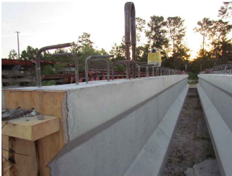
Figure 18 Laser machine at top of the girder
