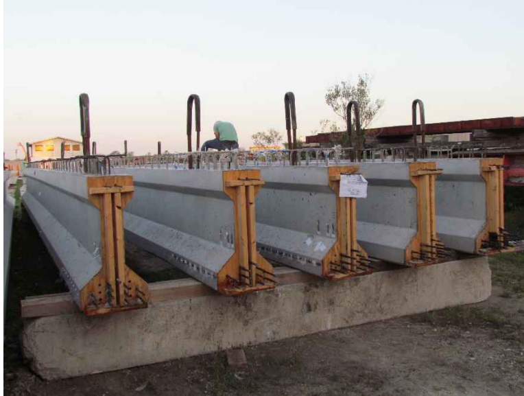
Figure 17 Girders at the casting yard
