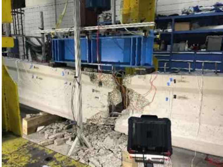
Figure 6-14 Crushing of concrete failure mode (Girder B3)
