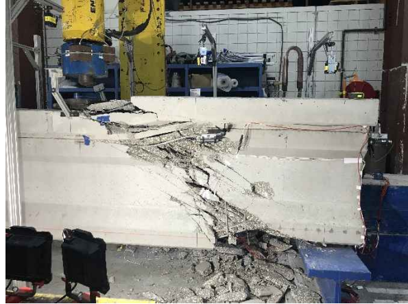
Figure 10-32 Web shear failure of Girder B3_2
