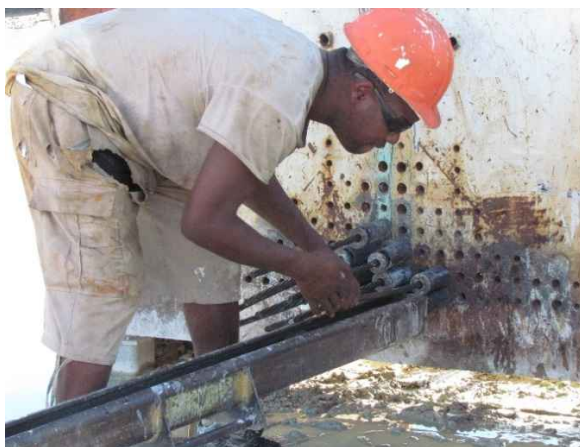
Figure 4-5 Seated stainless strands in the chucks
