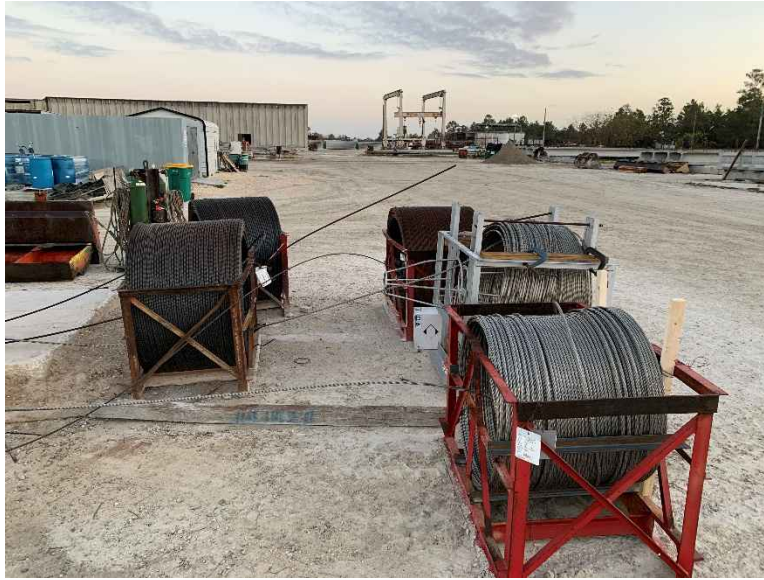
Figure 4-26 Stainless steel and carbon steel spools
