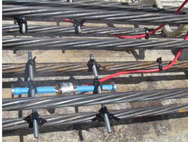
Figure 6-6 VWSG attached to the bottom layer of strands in Girder A2
