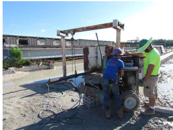
Figure 4-4 Monitoring applied force on electronic cell
