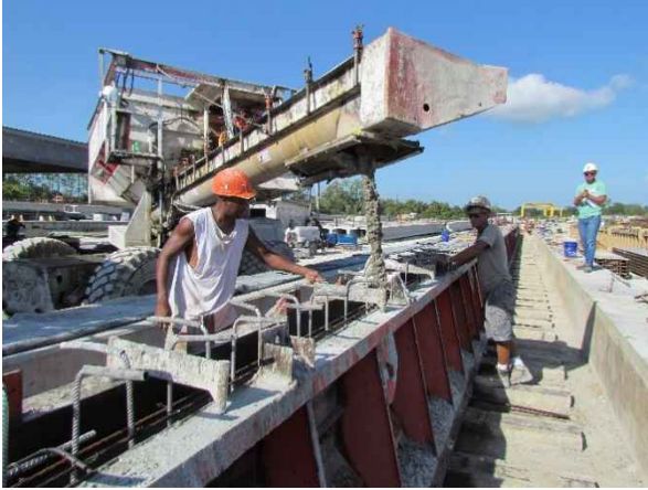
Figure 4-12 Casting concrete
