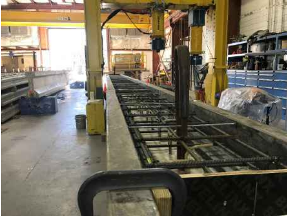
Figure 4-19 Girder before casting deck slab
