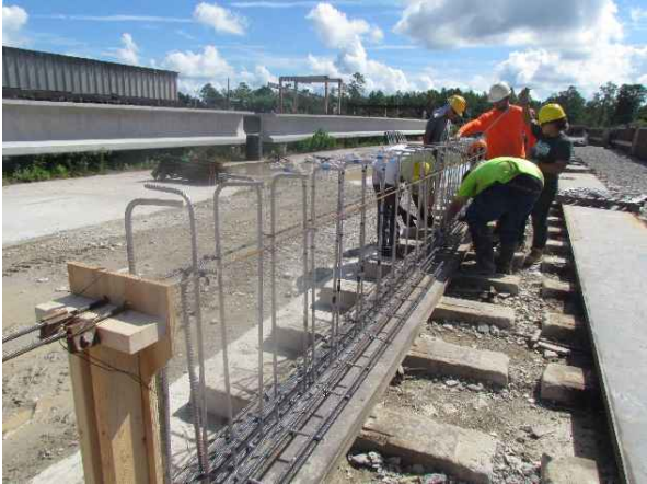
Figure 4-8 Tying stainless steel stirrups
