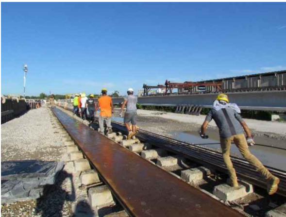
Figure 4-3 Running cables in the bed
