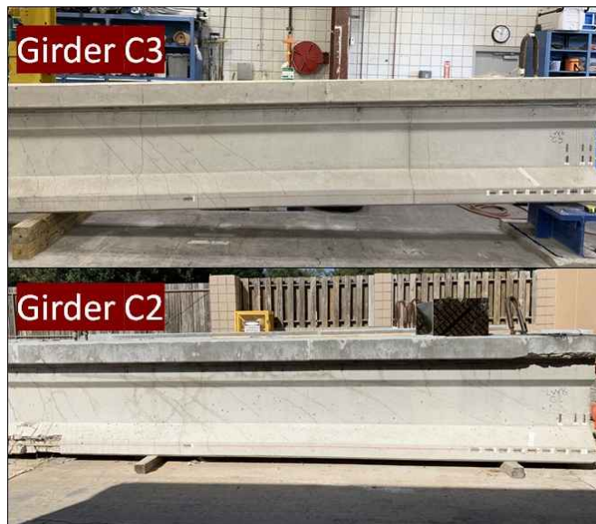
Figure 6-13 Crack patterns at ultimate load for Girder C2 and Girder C3
