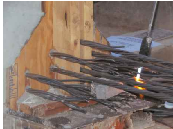
Figure 4-15 Releasing stainless steel strands using flame
