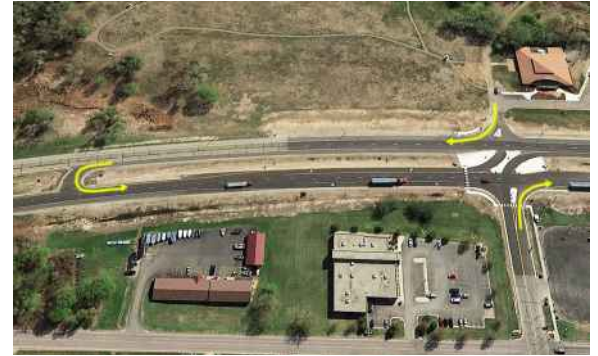
At this RCUT intersection (right), cars on the minor road must turn right and then use a U-turn lane (left) to complete a left turn or go straight across. A matching U-turn further to the right is not shown.
