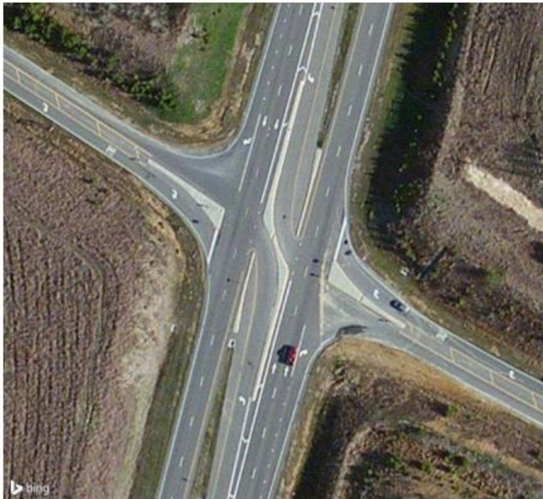
Stop-controlled RCUT intersection on US-1 near Southern Pines, NC.
