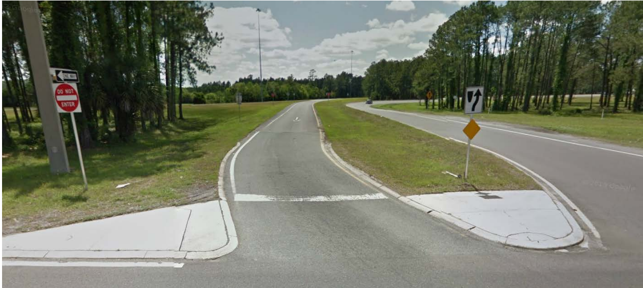
Figure 7. Entrance and exit ramps at a partial cloverleaf interchange, exit 343 on I-10. The Do Not Enter sign is located some distance from the exit ramp and may not be illuminated by drivers' headlights.
