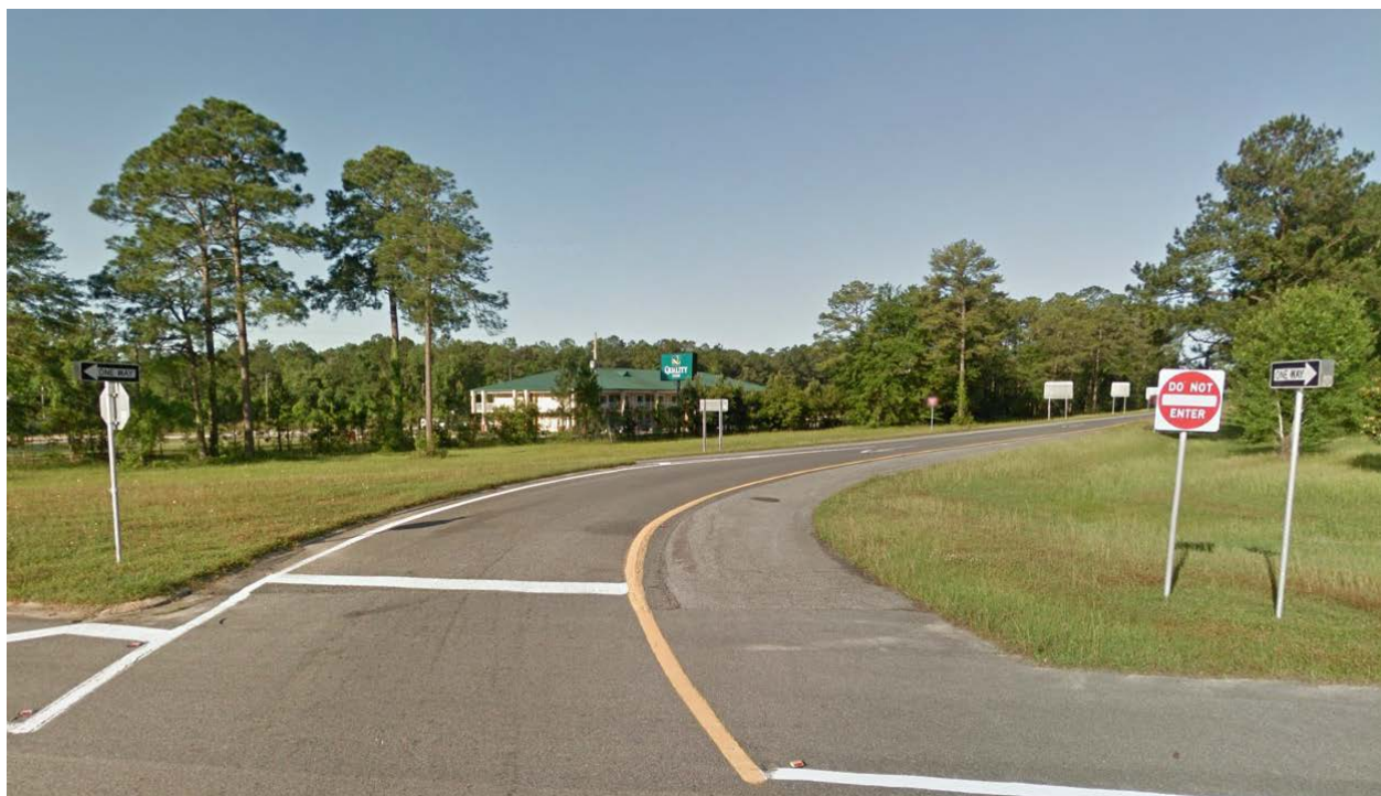
Figure 5. A stop bar painted at the terminal of the entrance ramp provides a cue that cars are likely to be approaching from the opposite direction.
