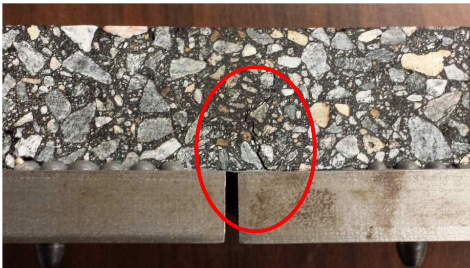
Figure 3.10. Specimen Cracking after the OT
