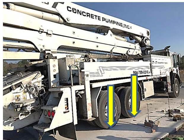
Figure 7.3: Concrete pump truck loading precast panels
