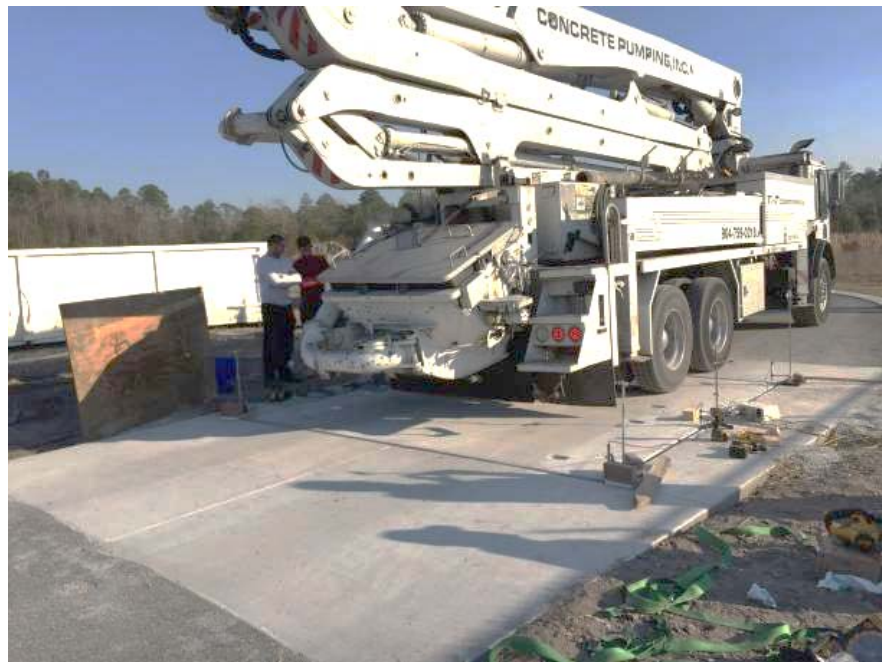
Figure 8.16: Allowing vehicles on the temporary precast panels
