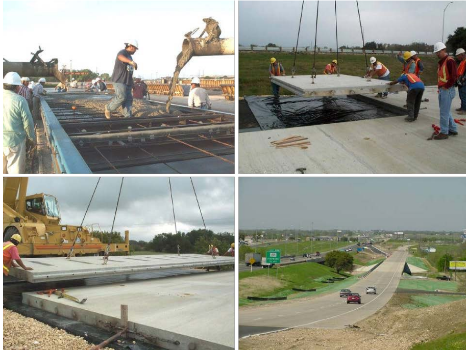
Figure 2.10: Precast pavement construction
