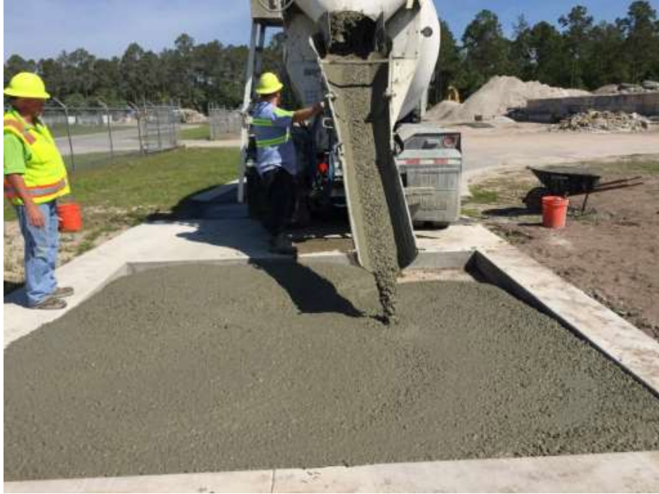
Figure 8.23: Replacement slab casting with SCC mix
