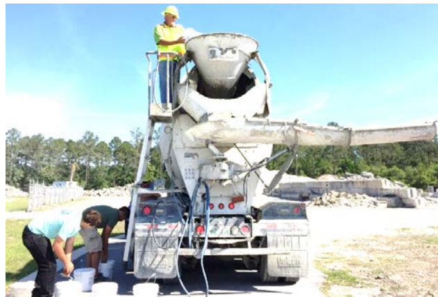
Figure 6.22: Addition of the accelerator at the track
