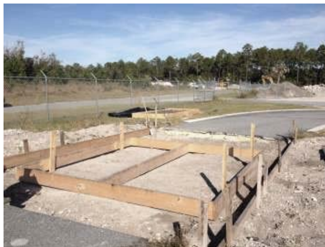
Figure 6.2: Preparing forms for the replacement-slab test-pit
