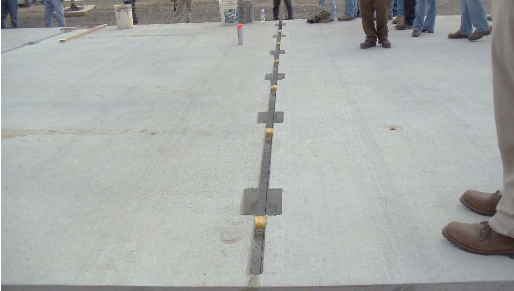
Figure 2.13: Joint and posttensioning ducts between adjacent panels
