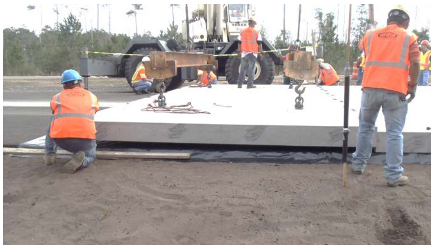
Figure 2.12: Installation of precast slabs on US 92
