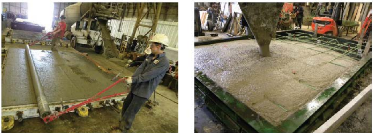
Figure 2.16: SCC placement and finishing of precast slabs
