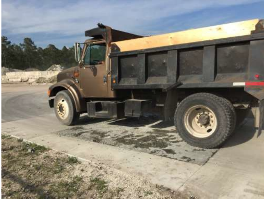
Figure 8.25: Allowing traffic on replacement slab after reaching required strength
