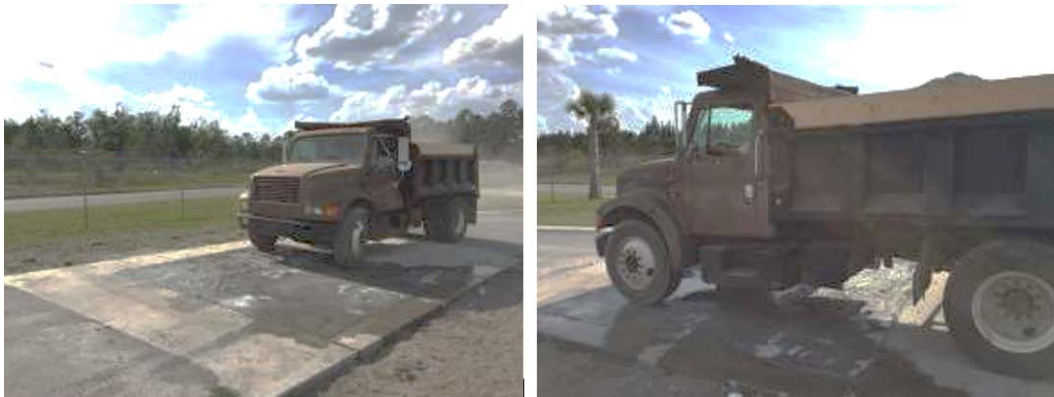
Figure 6.26: Load testing of the replacement slab using a 25,000 lb truck
