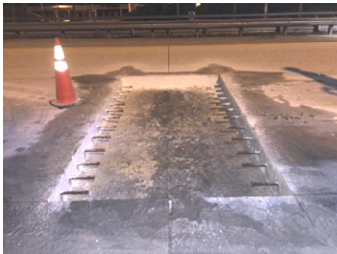
Figure 8.20: Replacement slab pit ready for concrete placement
