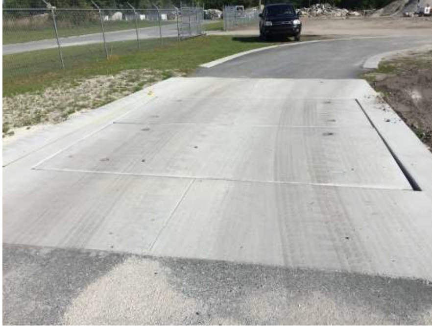
Figure 8.15: Two precast panels temporarily filling a 12' x 12' x 8" slab replacement pit
