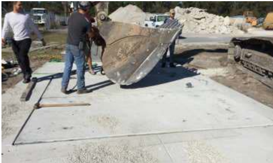
Figure 6.15: Placement of the two precast panels
