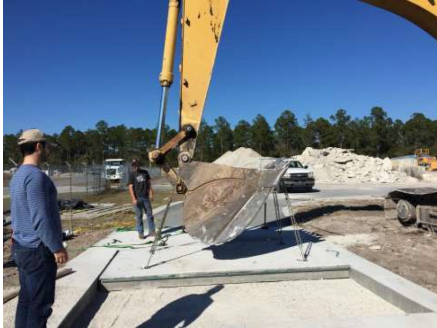
Figure 8.13: Installation of the first precast panel using a backhoe
