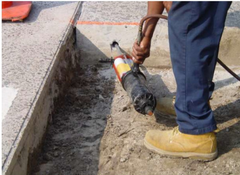
Figure 8.18: Application of epoxy starting from the back of the hole
