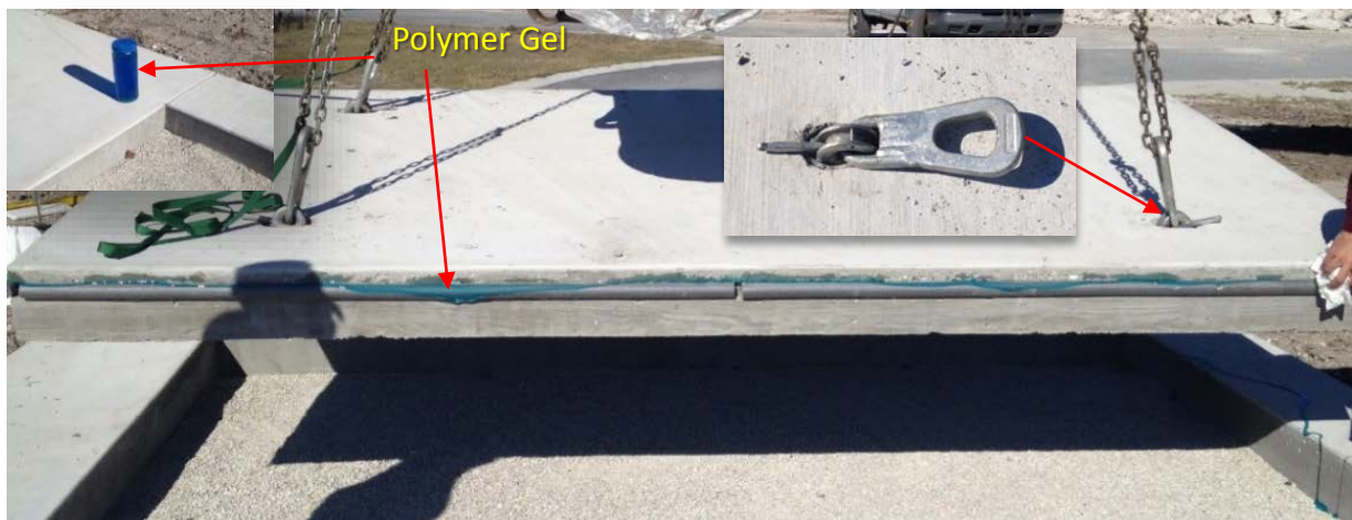
Figure 6.11: Lubricated backer rod
