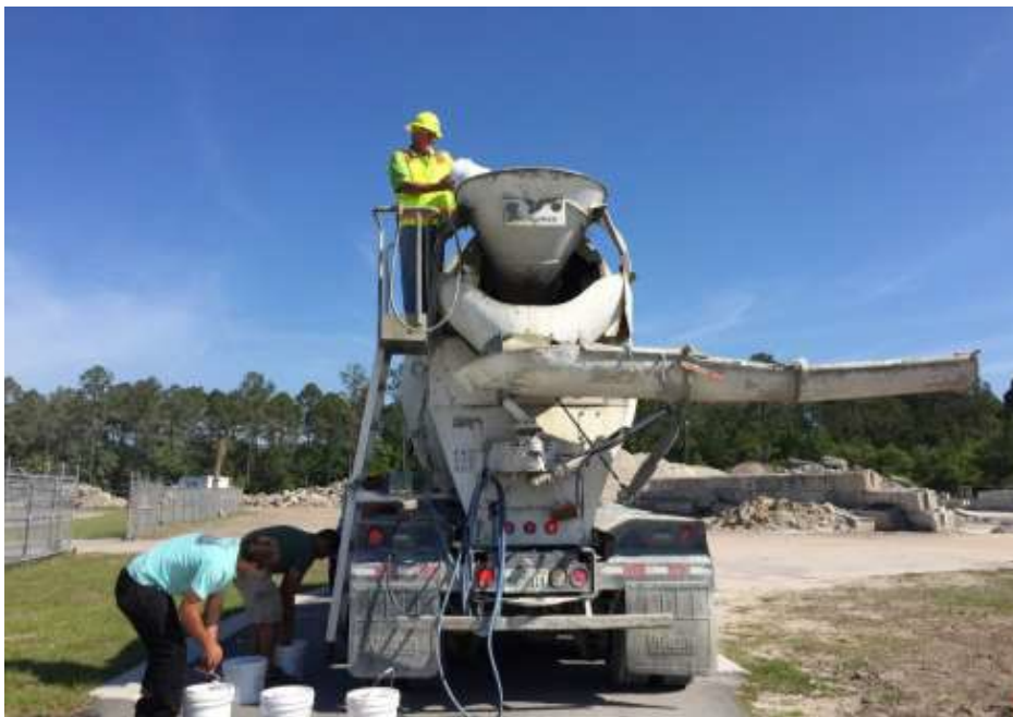
Figure 8.22: Add accelerator to the SCC mix at the jobsite
