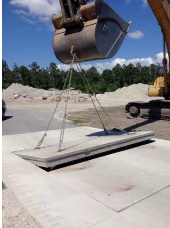
Figure 8.17: Removing temporary precast panels from the replacement pit
