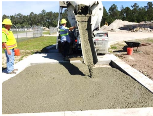
Figure 6.23: Discharging SCC mix in the pit to cast the replacement slab
