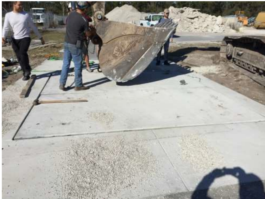
Figure 8.14: Installation of second panel
