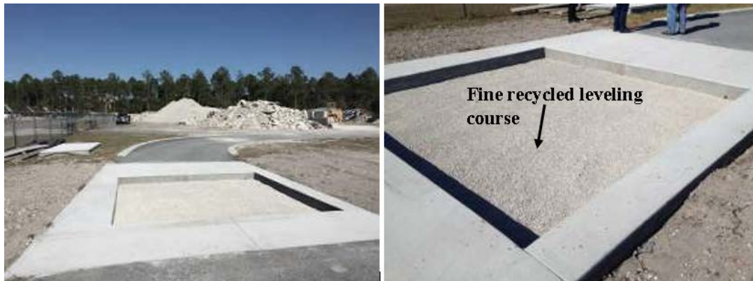
Figure 6.4: Test pit with fine recycled concrete aggregate as leveling course
