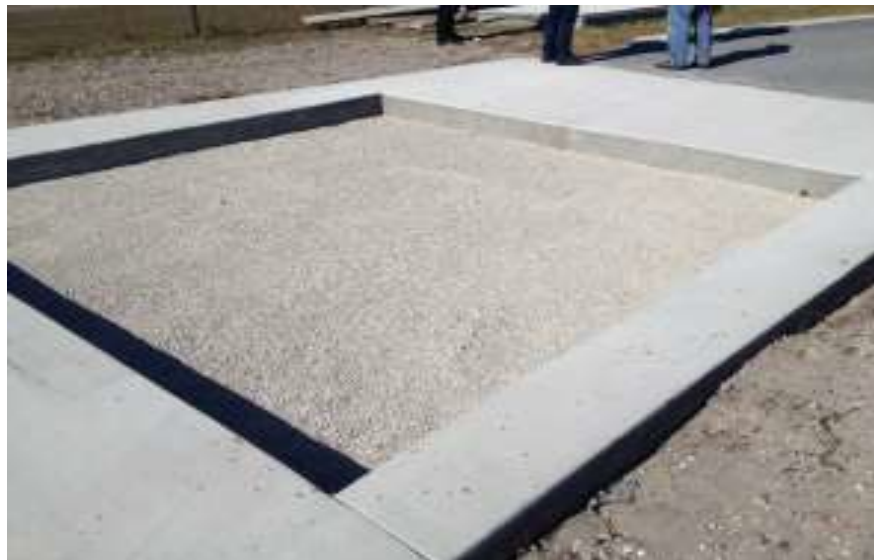
Figure 8.10: Fine recycled material for base leveling course
