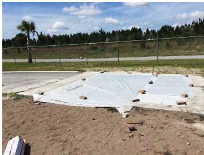
Figure 6.25: Slab curing with plastic sheet
