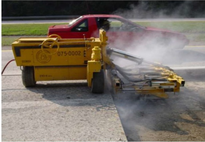
Figure 8.11: Drilling new holes for dowel bars with a Gang drill
