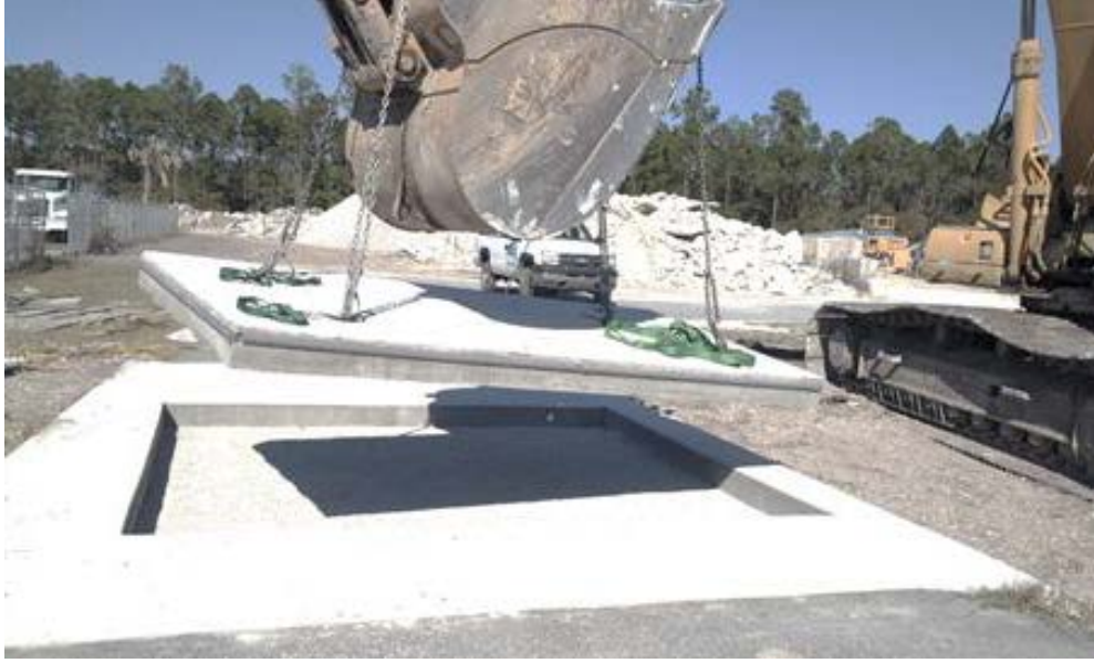
Figure 6.12: Rigging and maneuvering the precast panel
