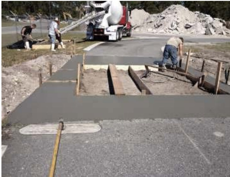
Figure 6.3: Paving concrete around the replacement slabs test pit
