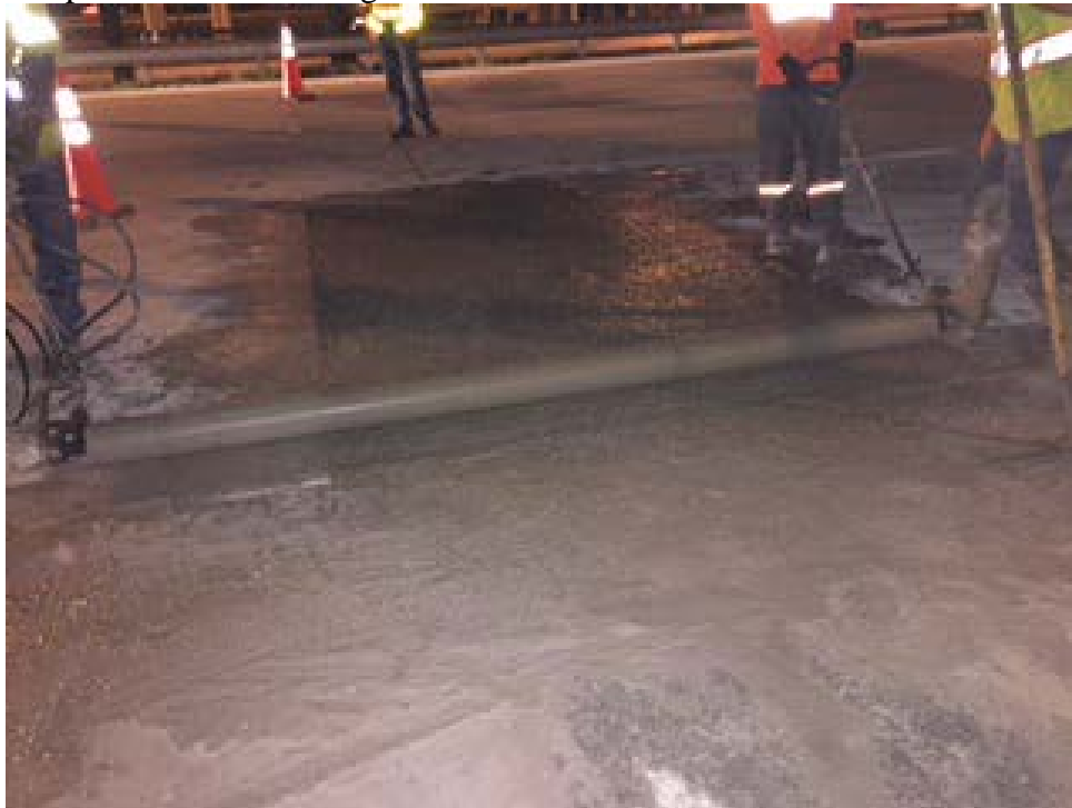
Figure 8.24: Final surface finish with Roller screed
