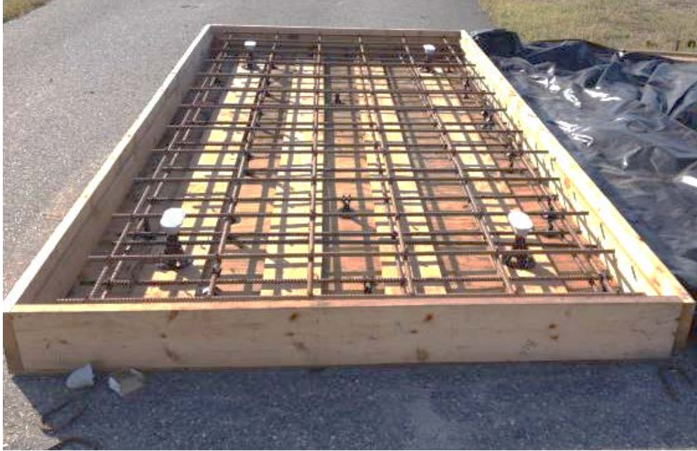
Figure 8.7: Reinforcement and form design
