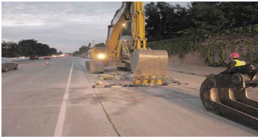
Figure 2.17: Removal of deteriorated concrete and formation of a replacement slab pit
