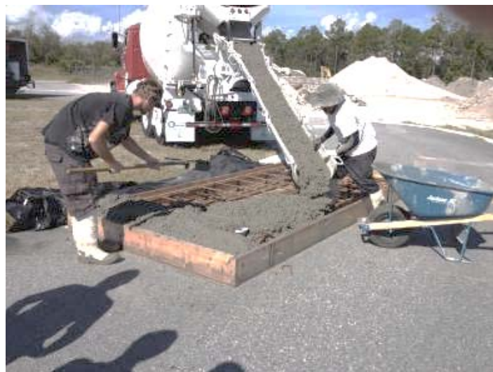
Figure 6.9: Casting of precast panel
