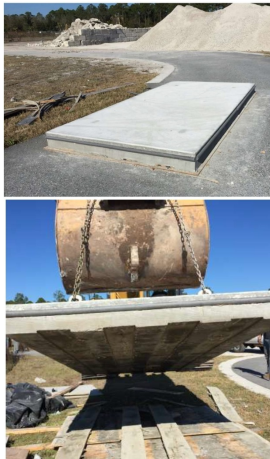
Figure 8.9: Demonstration panels showing backer rod and bottom recessed stripes
