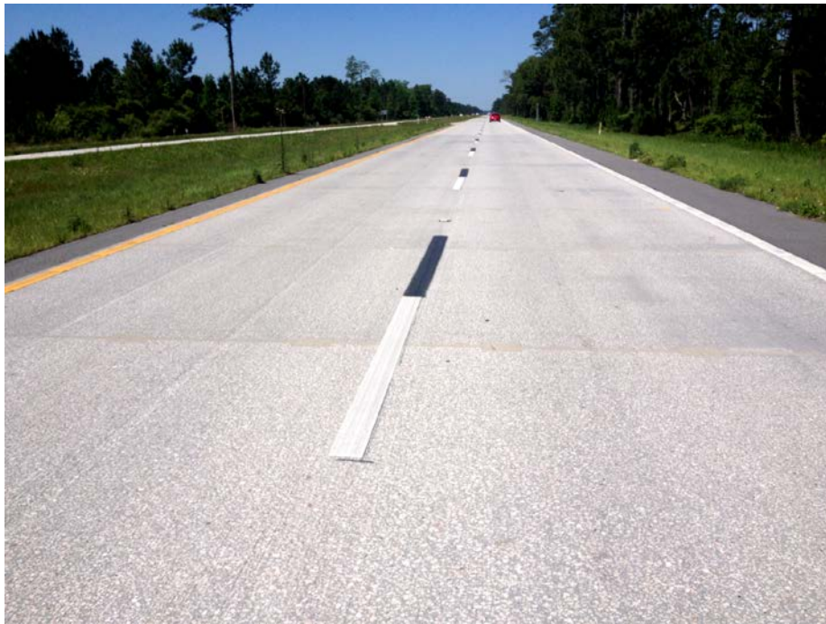
Figure 2.14: Project under traffic. Note joint grout and ground pavement surface
