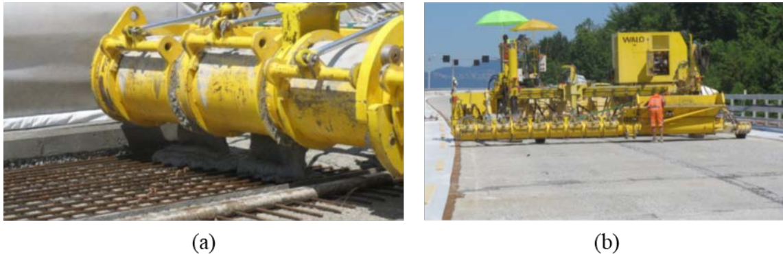
Figure 2.44: Cast-in-place UHPC overlay, immediately (a) before and (b) after placement [31]
