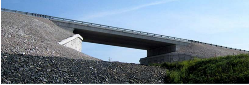
Figure 2.5: Hawk Lake Bridge [5]
