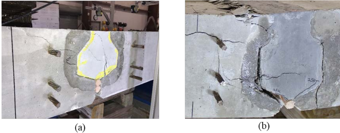
Figure 5.67: (a) Failed 12A1-1 specimen and (b) Failed 12A2-1 specimen
