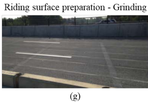
Figure 2.43: General procedure for mixing and casting UHPC [31]
