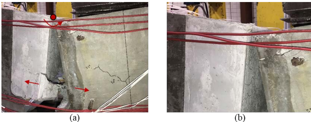
Figure D.9: 18F1-1: (a) failed specimen and (b) close-up of hinge developing in top corner of precast member next to UHPC joint
