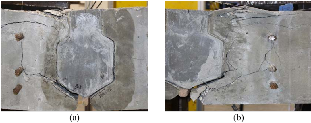
Figure D.55: 12A2-2: (a) west side failed specimen and (b) east side joint face showing similar rupture pattern with more amount of cracks
