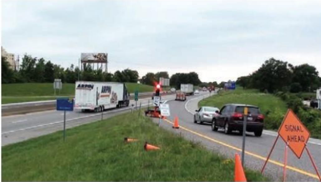
Figure 5.2: Temporary Ramp Metering Application in Missouri (Source: Sun et al., 2013)
