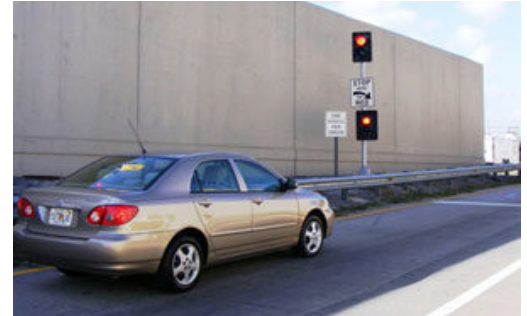
In a recent study, a Florida International University and University of North Florida research team developed guidelines for activating ramp meter signals during non-recurring congestion.
