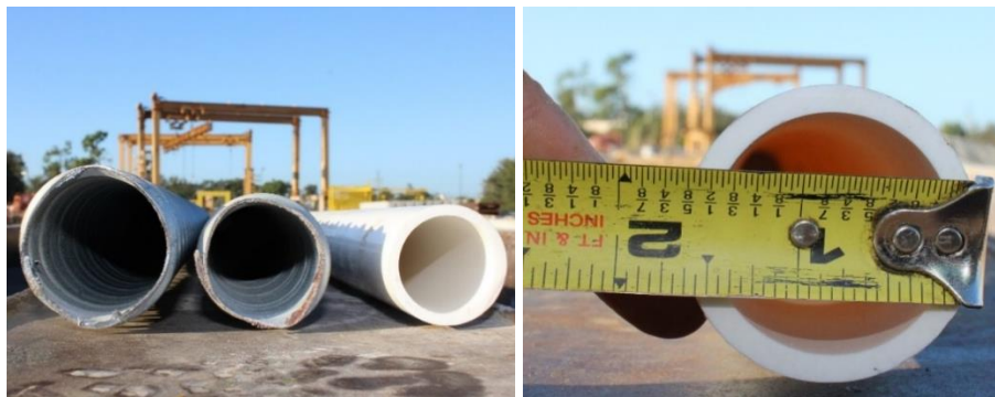
Figure 50: The pipes used for the construction
