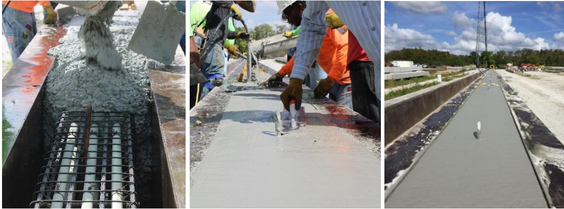
Figure 55: Casting concrete
