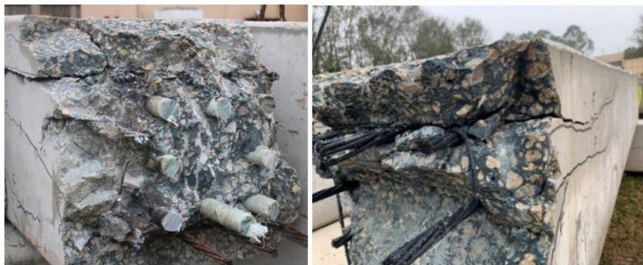
Figure 127: Two examples of the splitting cracks
