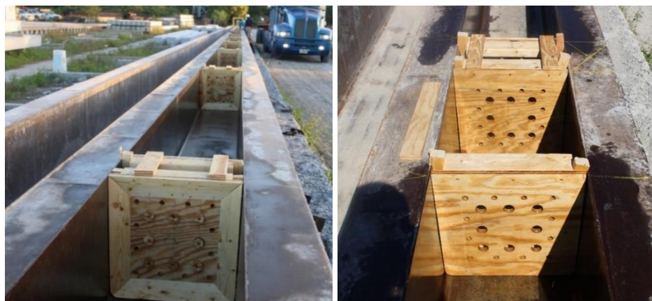
Figure 46: Wooden headers arrangement in casting bed
