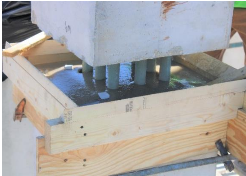
Figure 62: Filling the holes by epoxy and assembling pile specimens
