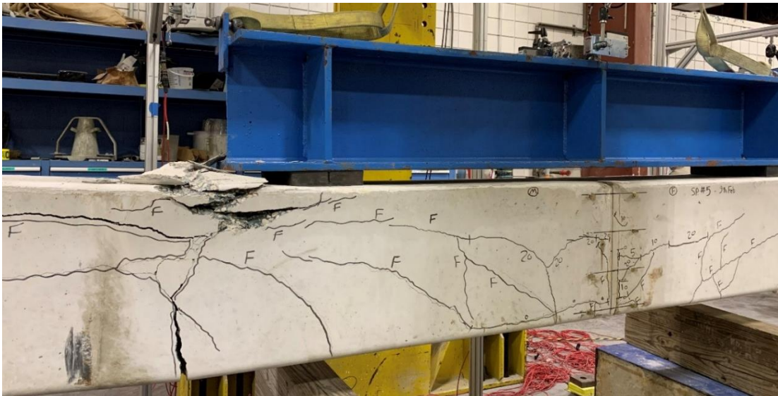
Figure 93: Crack propagation and failure mode of Specimen 5
