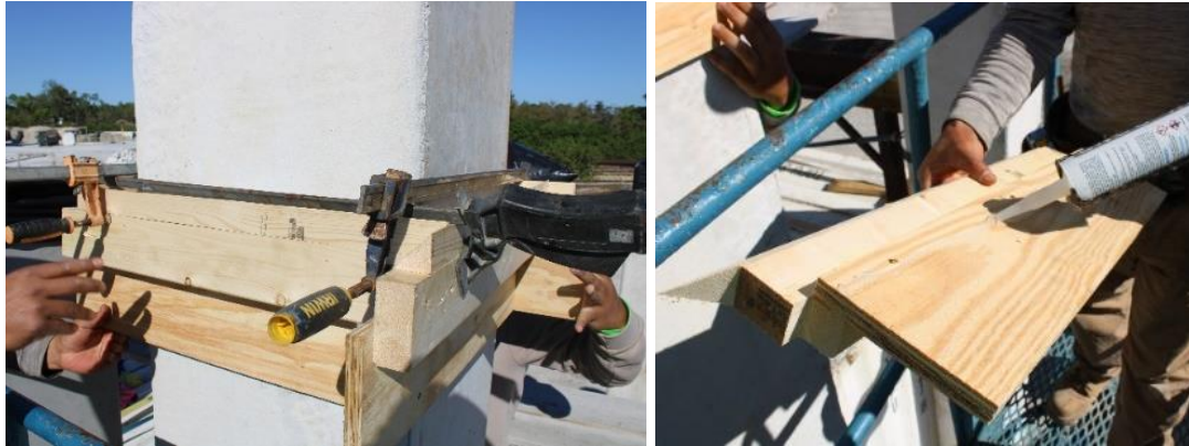
Figure 60: Wooden framework used for splicing the pile specimens
