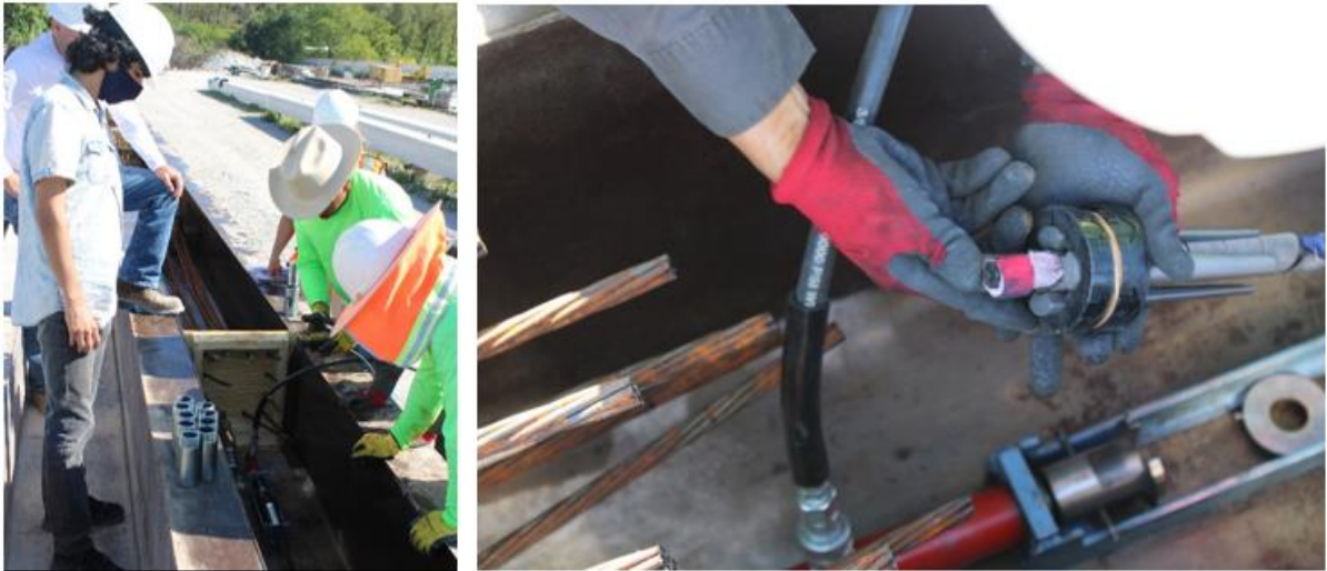
Figure 52: Coupling arrangement and installation by TRUSA
