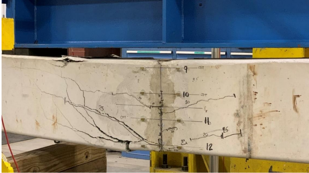
Figure 71: Crack propagation and failure mode of Specimen 1
