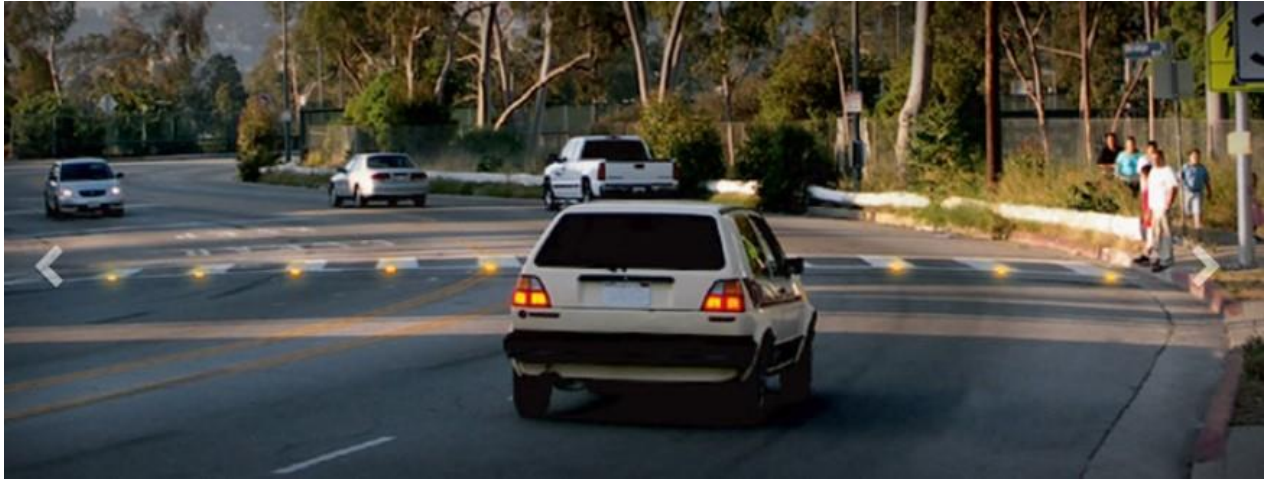
Figure 2-8: In-Roadway Warning Lights (Source: TAPCO, Inc., 2020)
