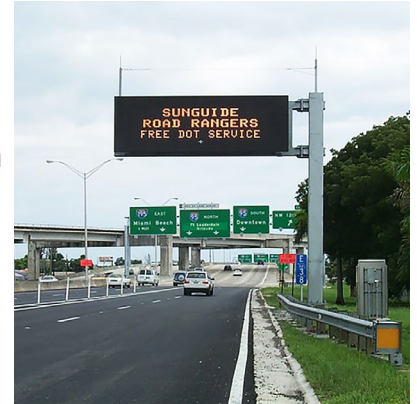
The dynamic message sign and other TSM&O strategies improve safety and traffic flow.
