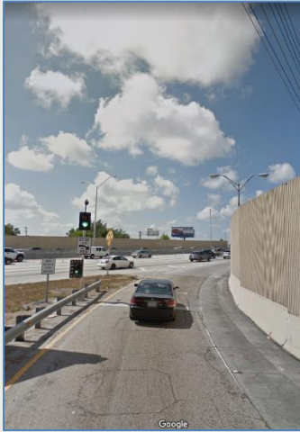
Ramp Metering Signal (RMS)
