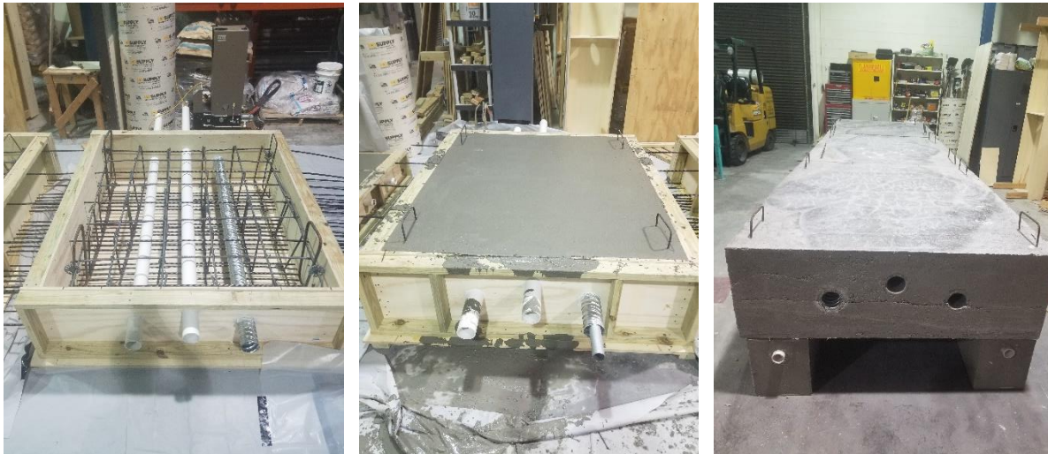
Figure 4-28: Construction of specimen.
