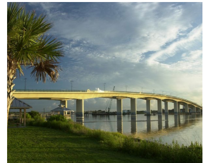
The Broadway Bridge in Daytona Beach is one of many made possible by post-tensioning.
