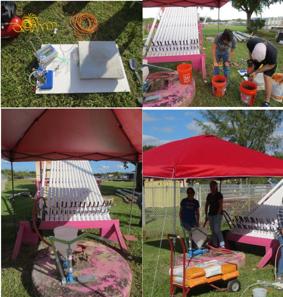
Figure 5.3. MIT grout mixing and injection
