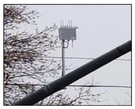
Figure 4-13 RSU Installed on Mast Arm (Leonard, 2002)
