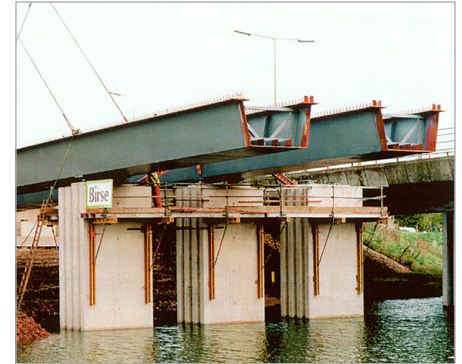
Box girders are placed during the construction of a bridge.
