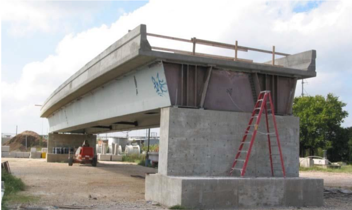
Figure 5-15. The University of Texas twin steel box girder bridge.
