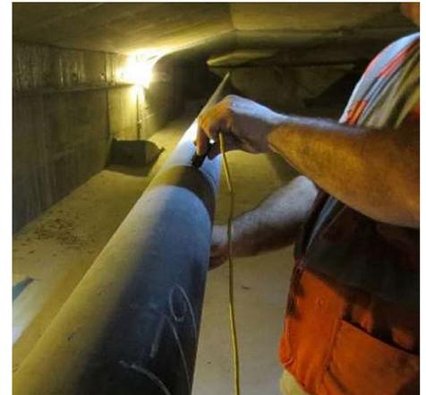
*A worker begins testing on a post-tensioning tendon inside one of the box girders that make up the Ringling Bridge.*
