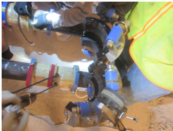
Figure 9. A steel outer shell being installed.
