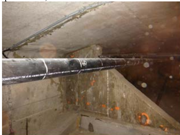
Photograph 3- Location station marks on duct
