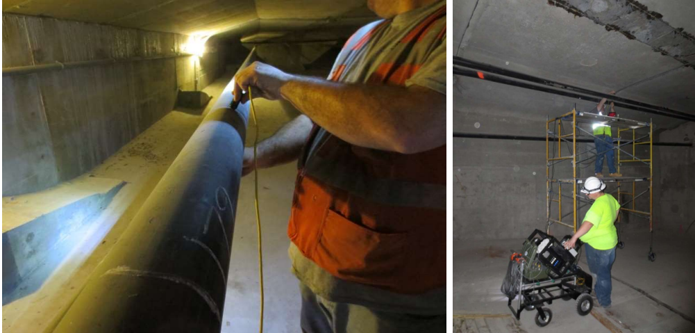
Figure 4-1: Ultrasonic/sonic testing on external PT tendons.
