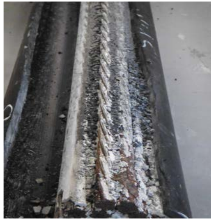
Photograph 6- Duct 36 with PVC Jacket Removed
