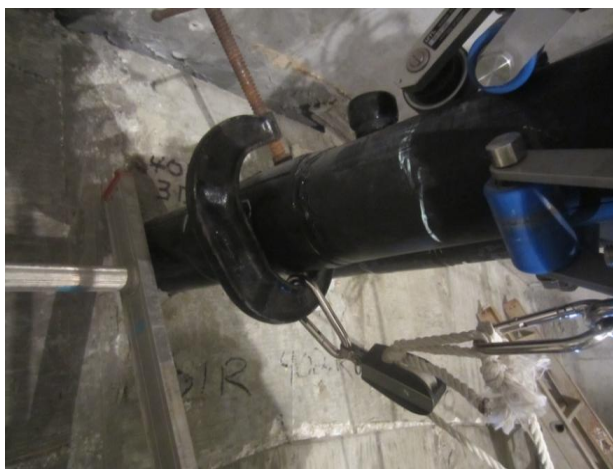
Figure 25. Installing a steel clamp and a pulley.
