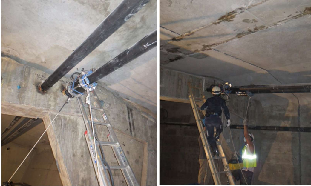
Figure 3-4: Scanning of tendons using MMFM.
