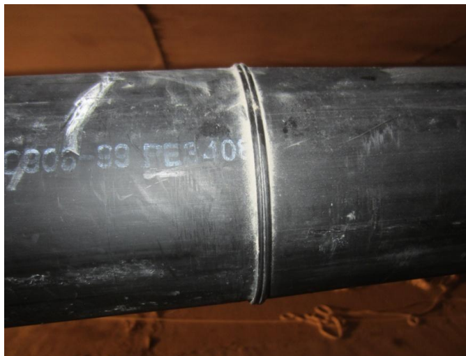
Figure 32. Extruded HDPE welding joint.
