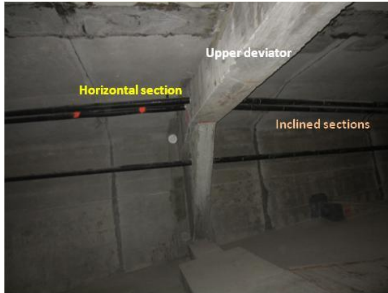
Figure 18. Tendons going through an upper deviator.
