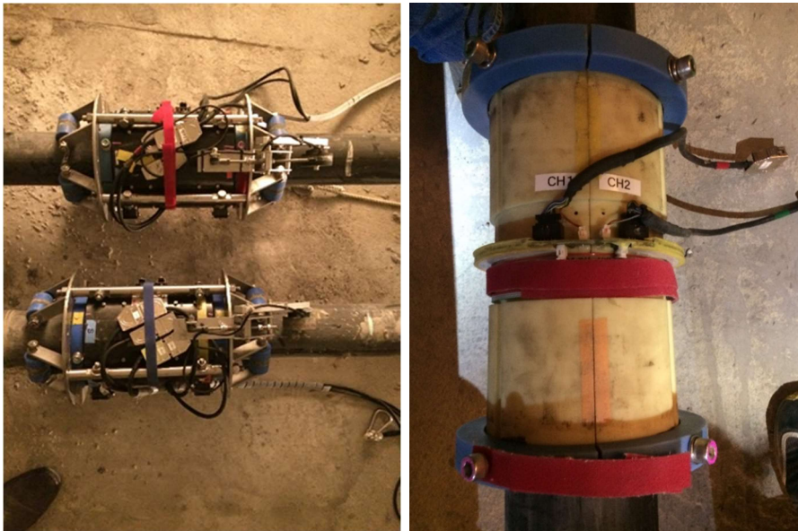
Figure 3-1: Installation of search coil and magnetizer on PT tendon.
