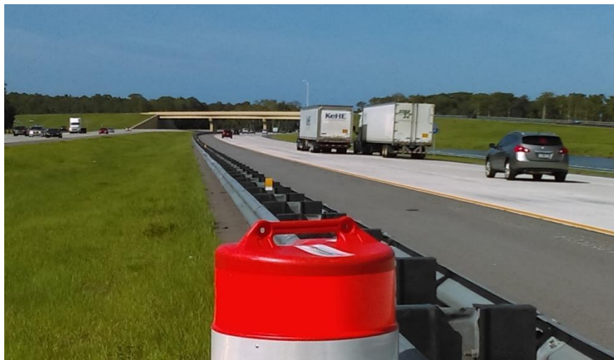
Figure 3-6. iCone #1 Located Ahead of the Curve (and Upstream of Work Zone)
