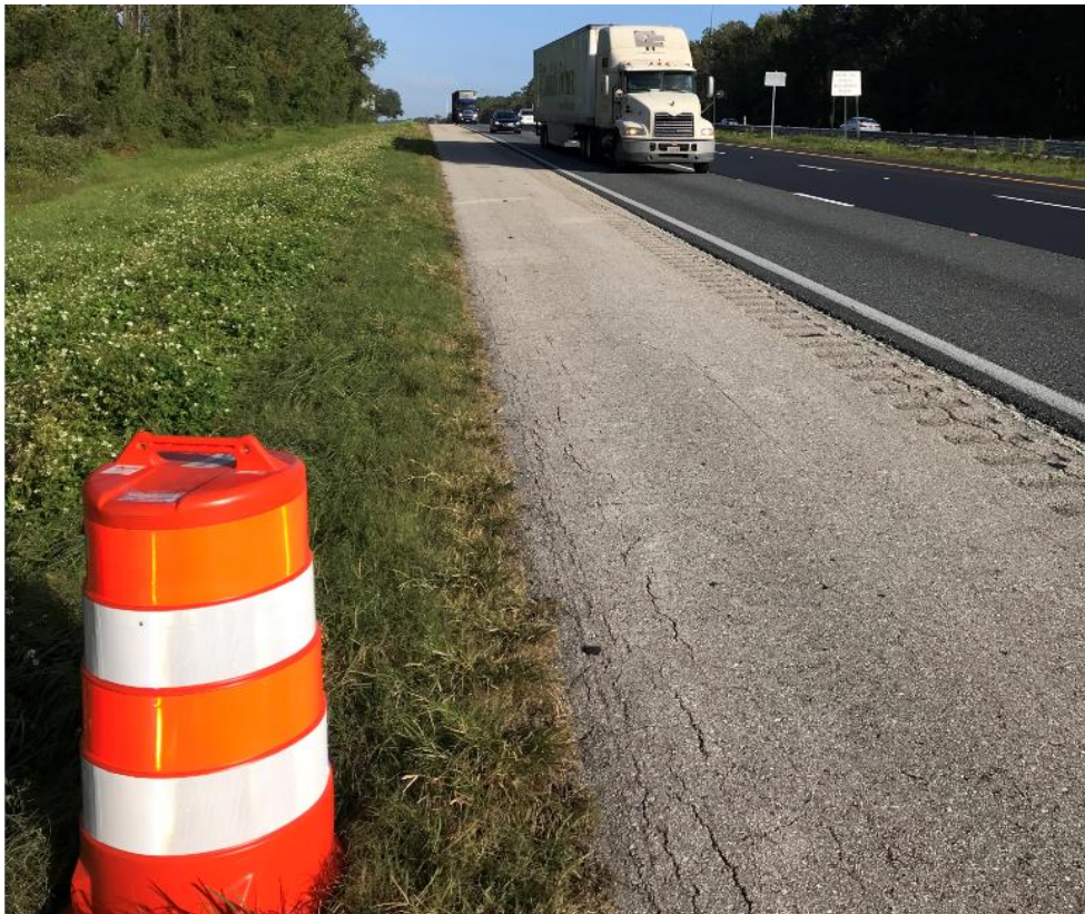
Figure 4-5. iCones Placed Next to the Outside Shoulder
