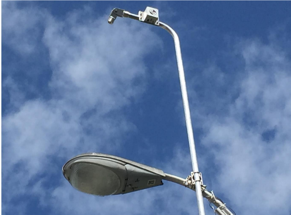
Figure 4-3. Adding Extension Structure to Increase Camera Height
