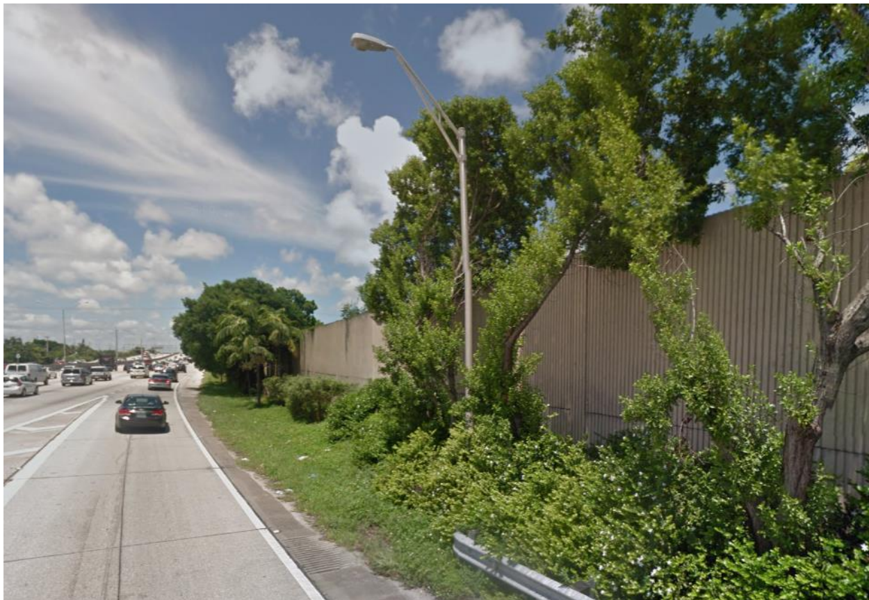
Figure 3-5. Potential Use of an Existing Light Pole at RMS #4 for Camera Installation
