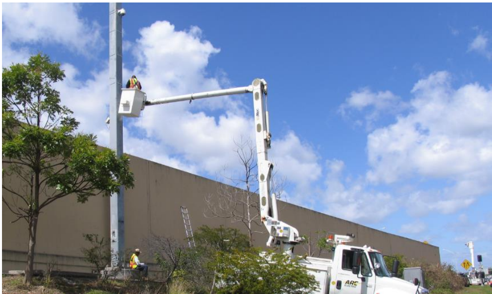
Figure 4-14. Installing Second FLIR Camera on FDOT Camera Pole
