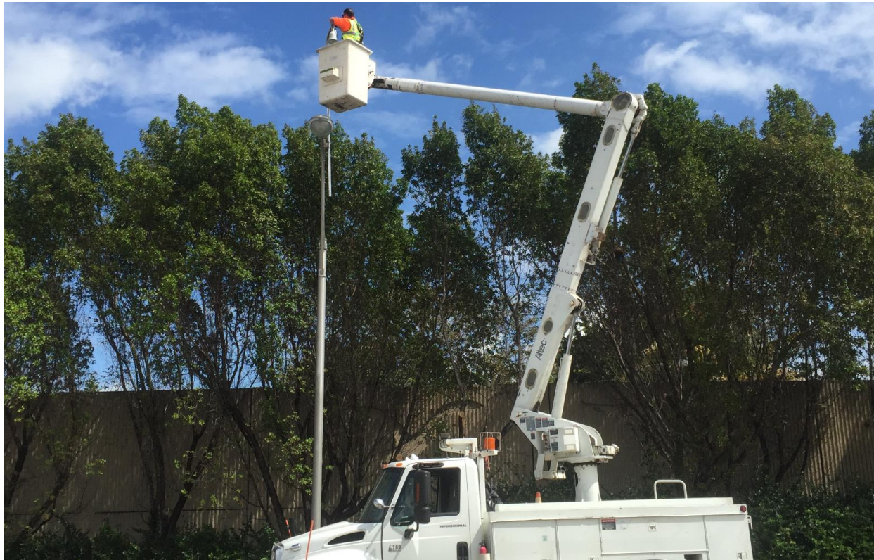
Figure 4-2. Installing GRIDSMART Camera on Light Pole
