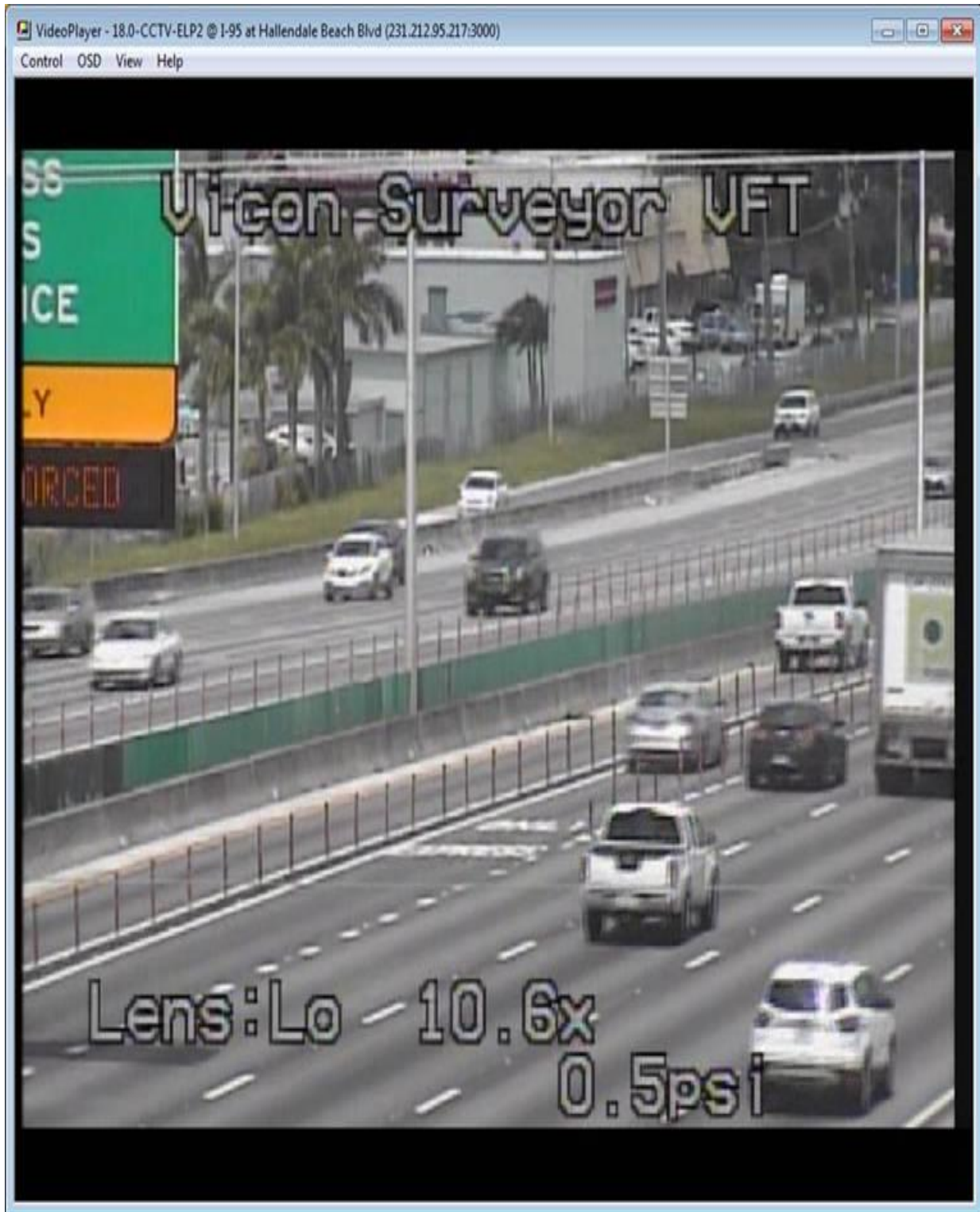
Figure 5: Asphalt Site 3—I-95 Express Lanes Northbound ramp from I-95 Mainline/Hallendale Beach Blvd (CCTV 18.0 ELP2)
