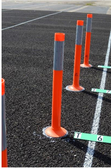
Figure 3.54. 607531-02-4 Sample (Asphalt Surface).
