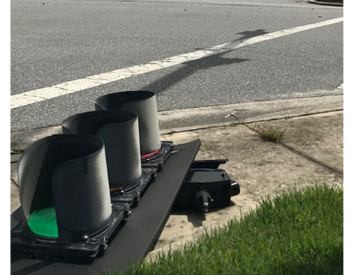
Downed traffic signals add to post-hurricane hazards and require significant repair.
