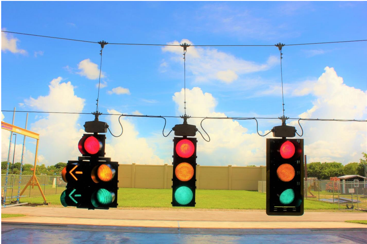
Figure 88: Damage after full range of wind speeds (damage to back plates and visors)
