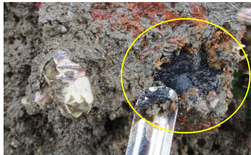
Figure 4.8. Example of Under Fouling Surface Condition.
