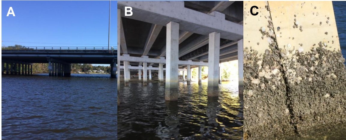
Figure 3.19. Images of US-301 Bridge over Alafia River (Site 4).
