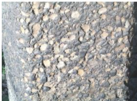
Figure 2.2. Microbial-induced Bio-deterioration of Concrete. (Trejo et al., 2008).
