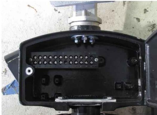
*Figure 197: Disconnect box after full test (wiring was removed)*
