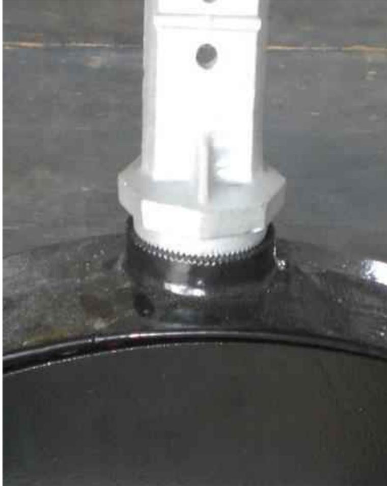
*Figure 30: Serrated teeth connection between the bracket and the top of the disconnect box with no noticeable damage*
