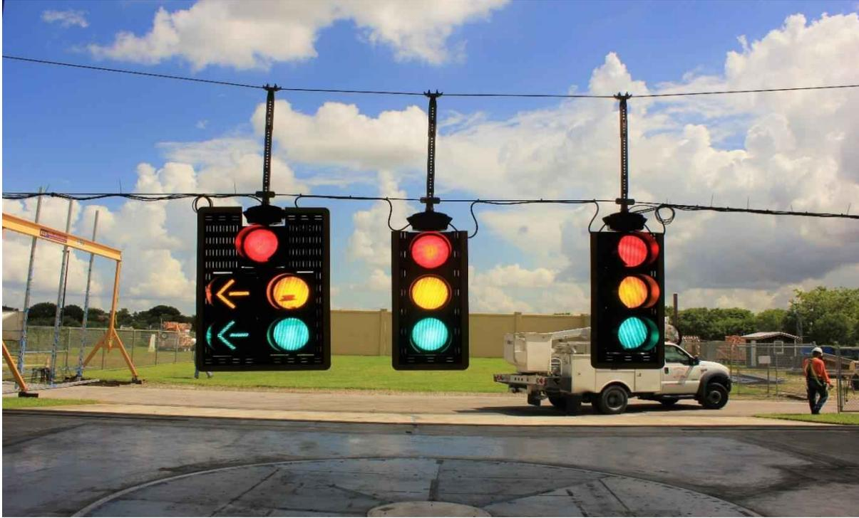
Figure 199: Traffic signals, hangers and span-wire
