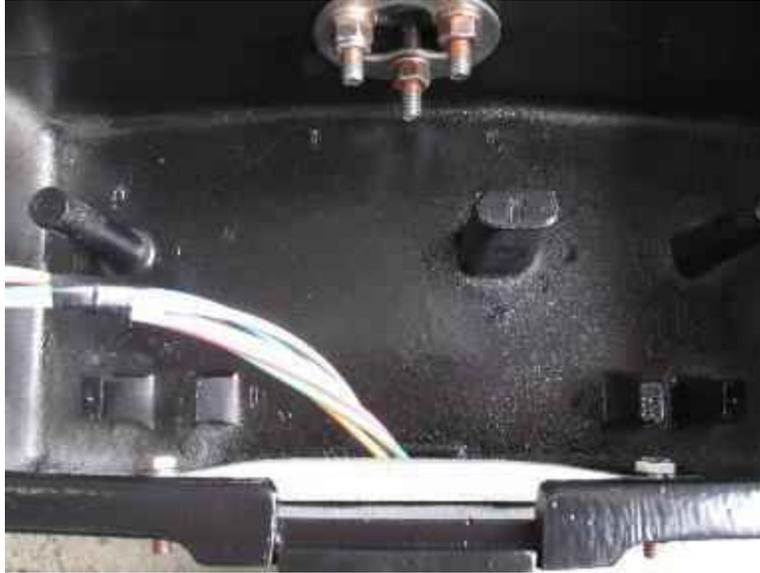
*Figure 98: Disconnect box for 3-section signal with no observed damage*
