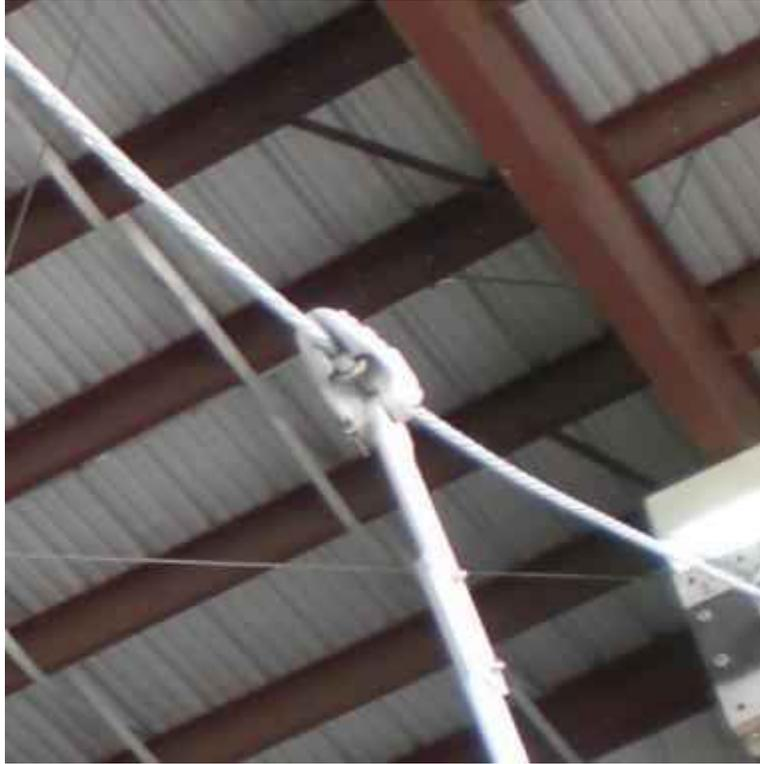
*Figure 34: Span wire clamp attached to the catenary cable with no noticeable damage*
