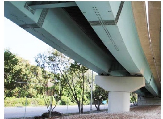
This view of one set of lanes on a Florida bridge shows the twin steel box girders and cross-braces.
