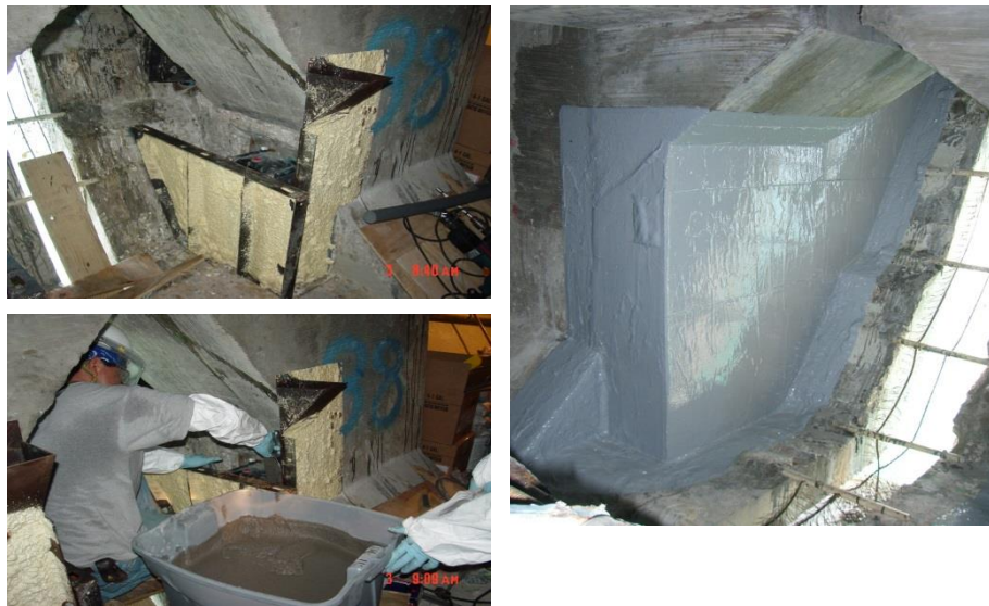
Figure 2-2: Epoxy pourback specimen design details (Hamilton and Alvarez, 2002)
